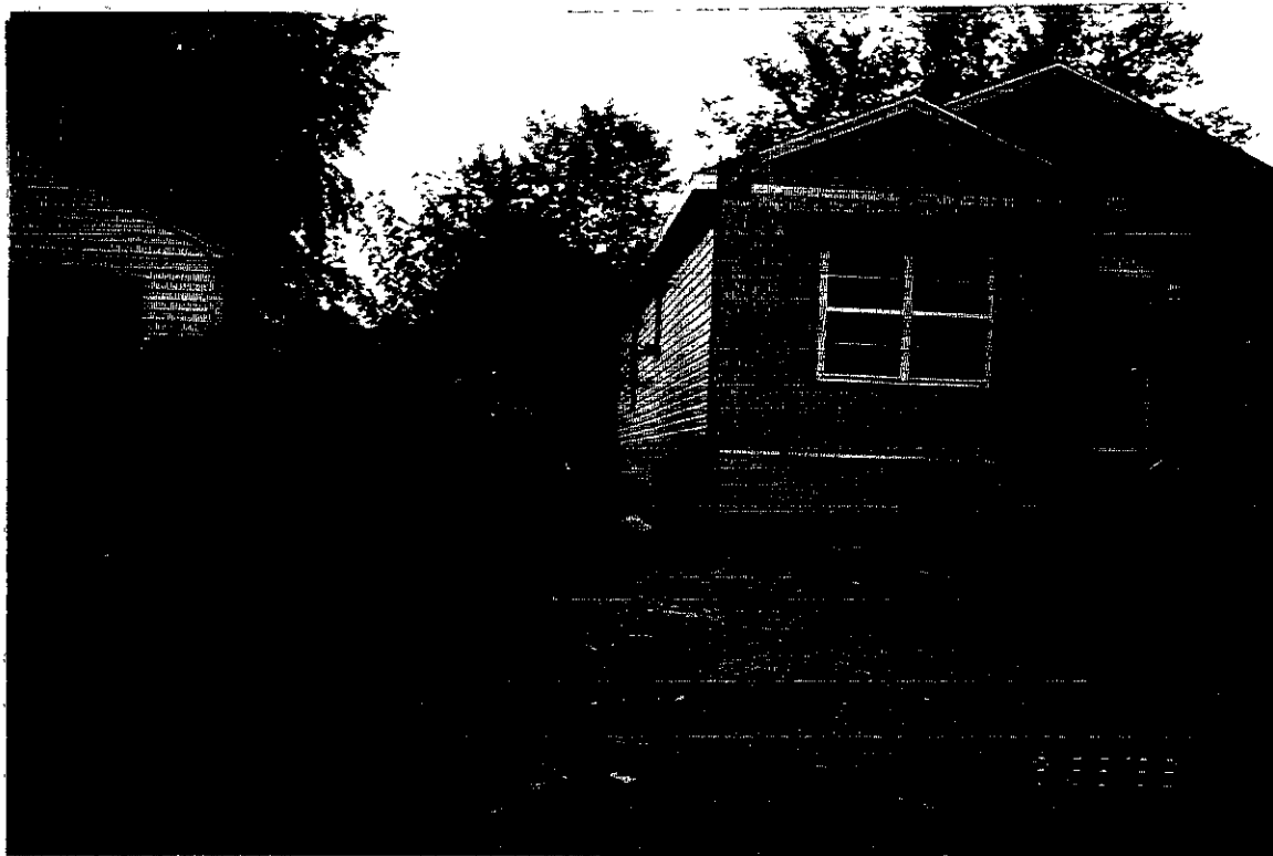
New home Construction on a 50 ft. wide lot. Gunpowder Rd.
