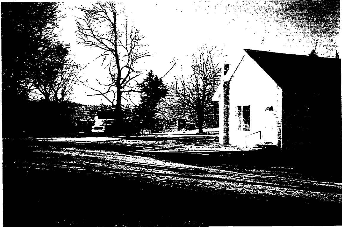
Rear of existing church Looking northwest, existing addition in foreground
