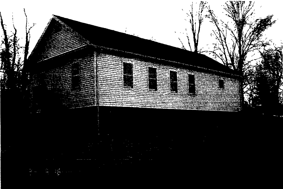
North side of existing Fellowship Hall Looking west
