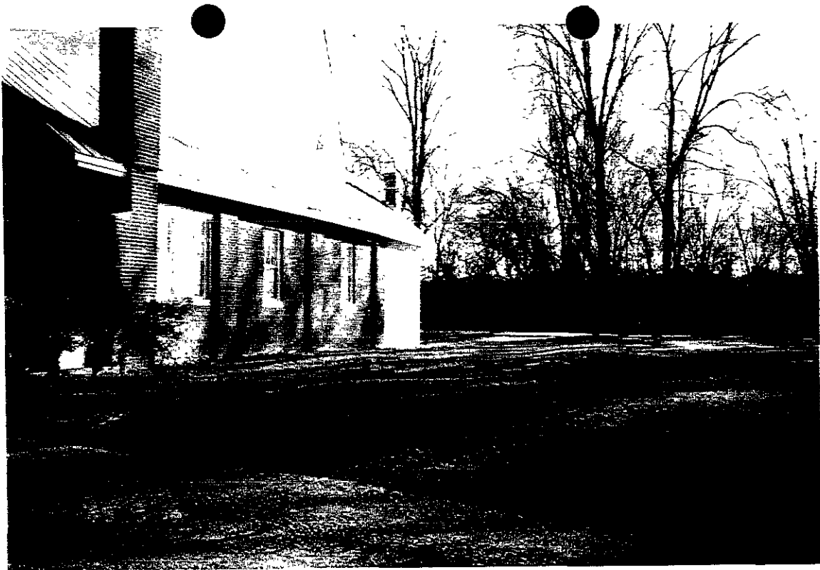
Southwest side of existing church Looking southeast
