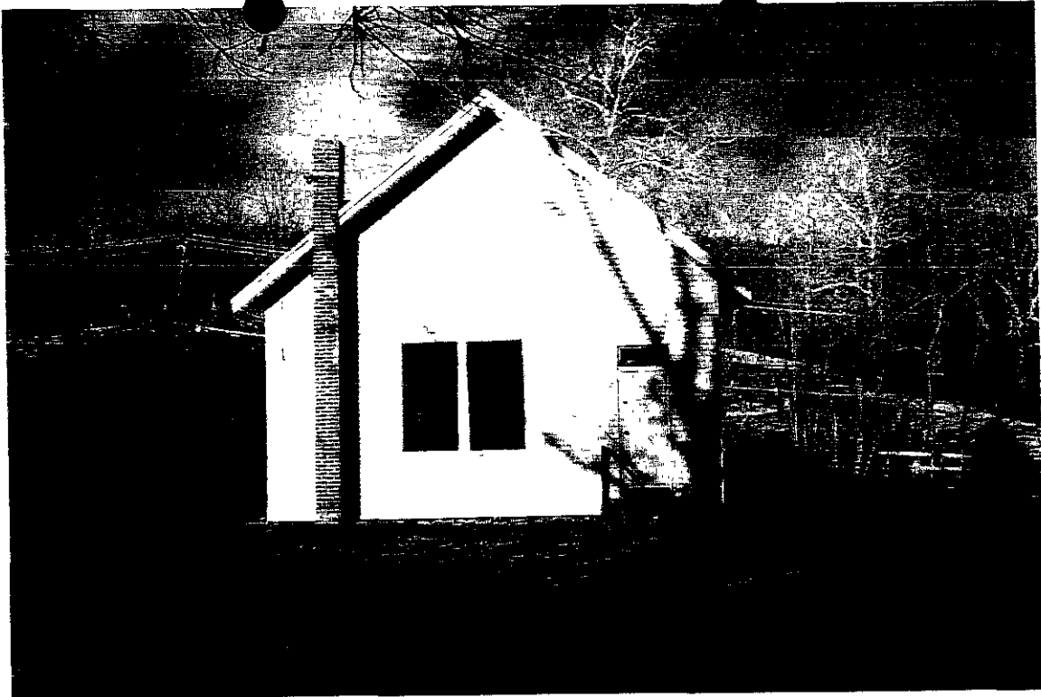
Rear of existing church Looking north, existing addition in foreground
