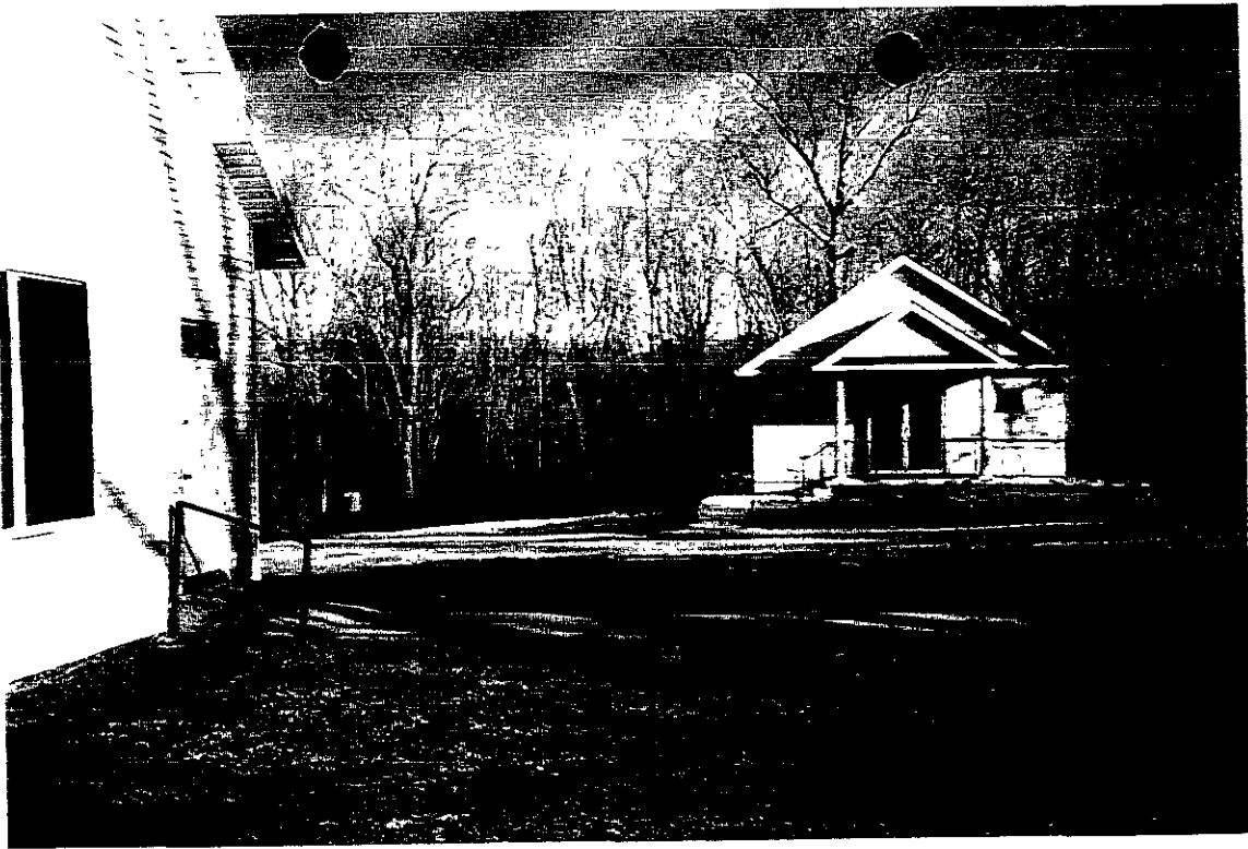
Existing Fellowship Hall Looking east, existing church in foreground
