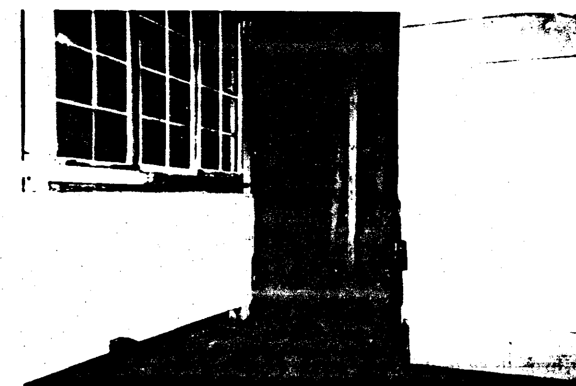
8. LOOKING AT BACK CORNER OF SUMMER KITCHEN (HOUSE) LARGE OPENING EXPOSED TO WEATHER FOR MANY YEARS - FLOOR & FOUNDATION GONE.
