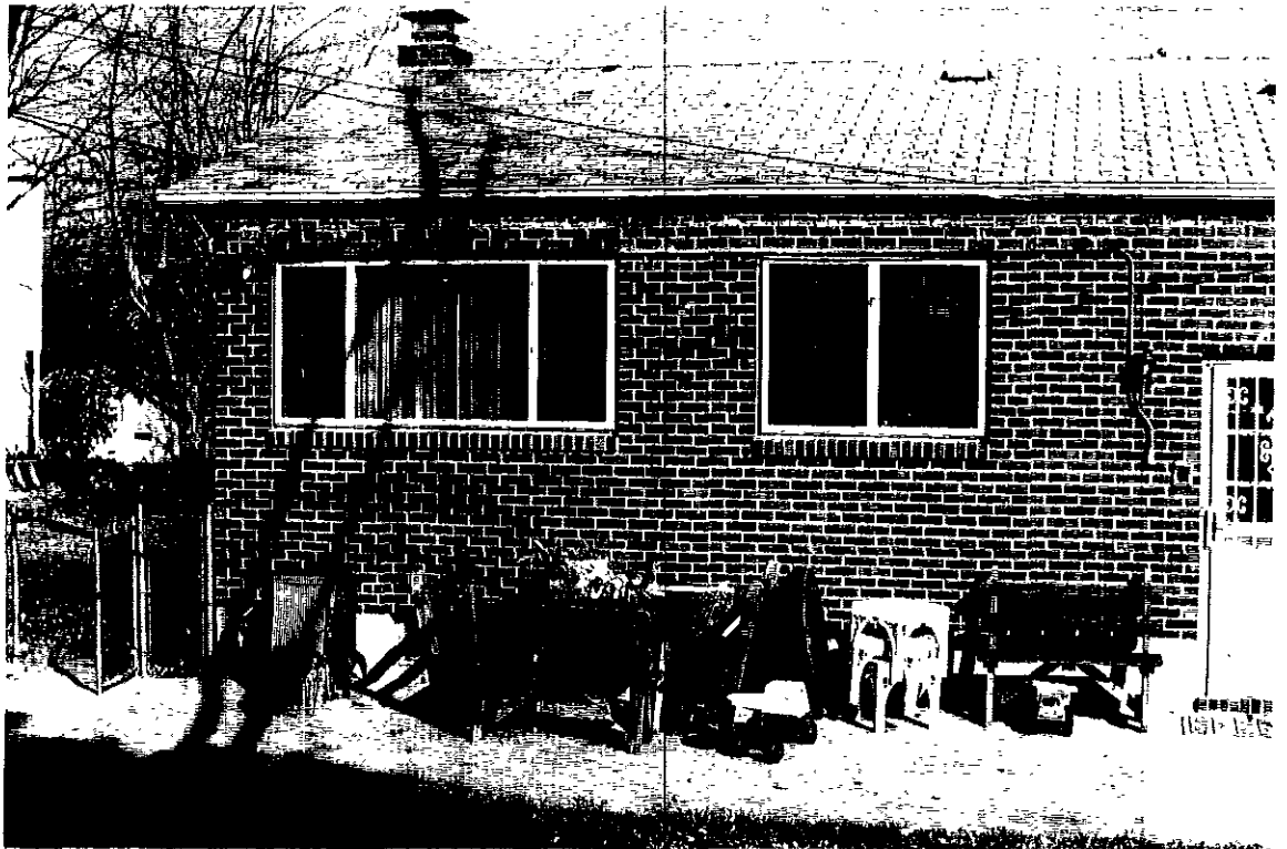
Rear of 5303 Dew Garth. Addition will extend across 20' out and out 10' (end of current concrete pad).
