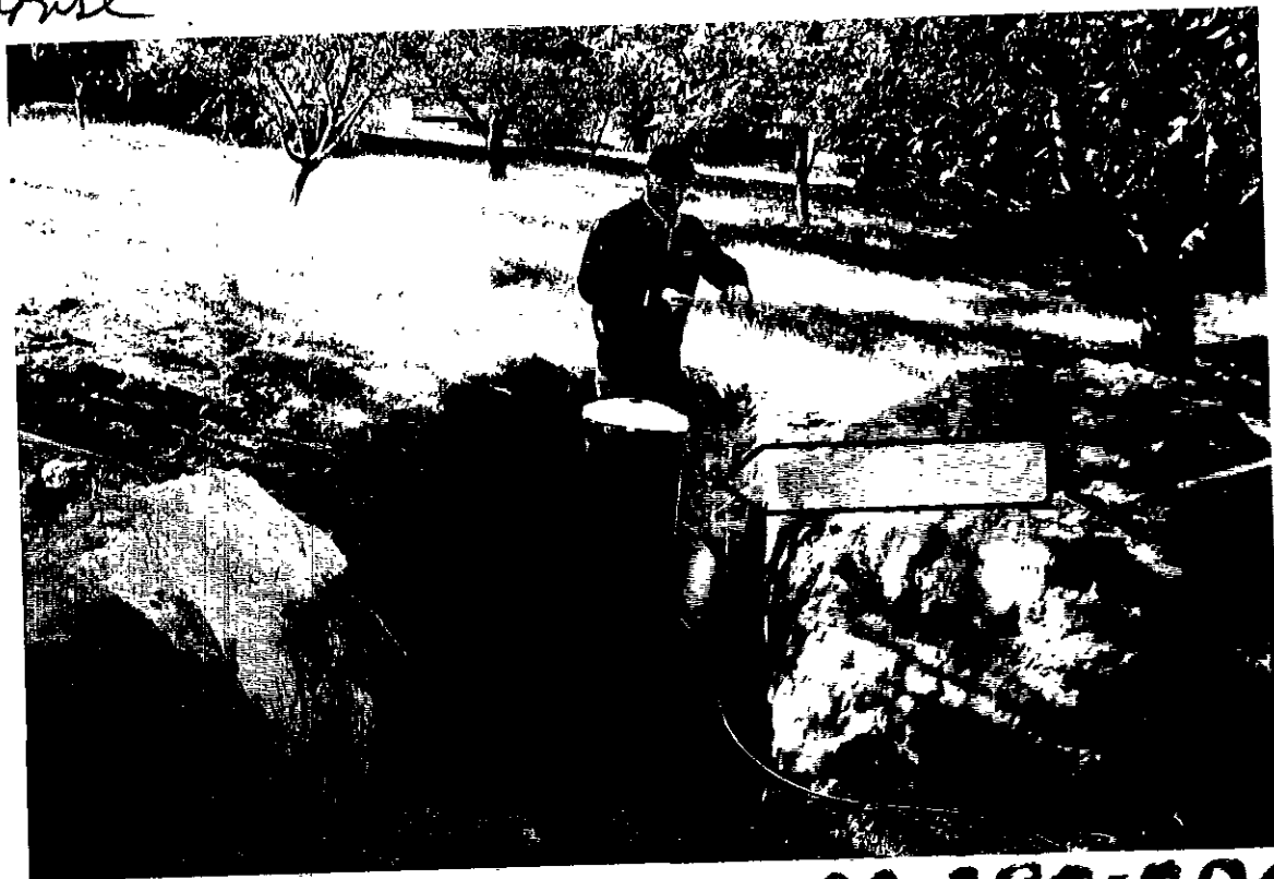
photo #2 propane Tank in Front yard
