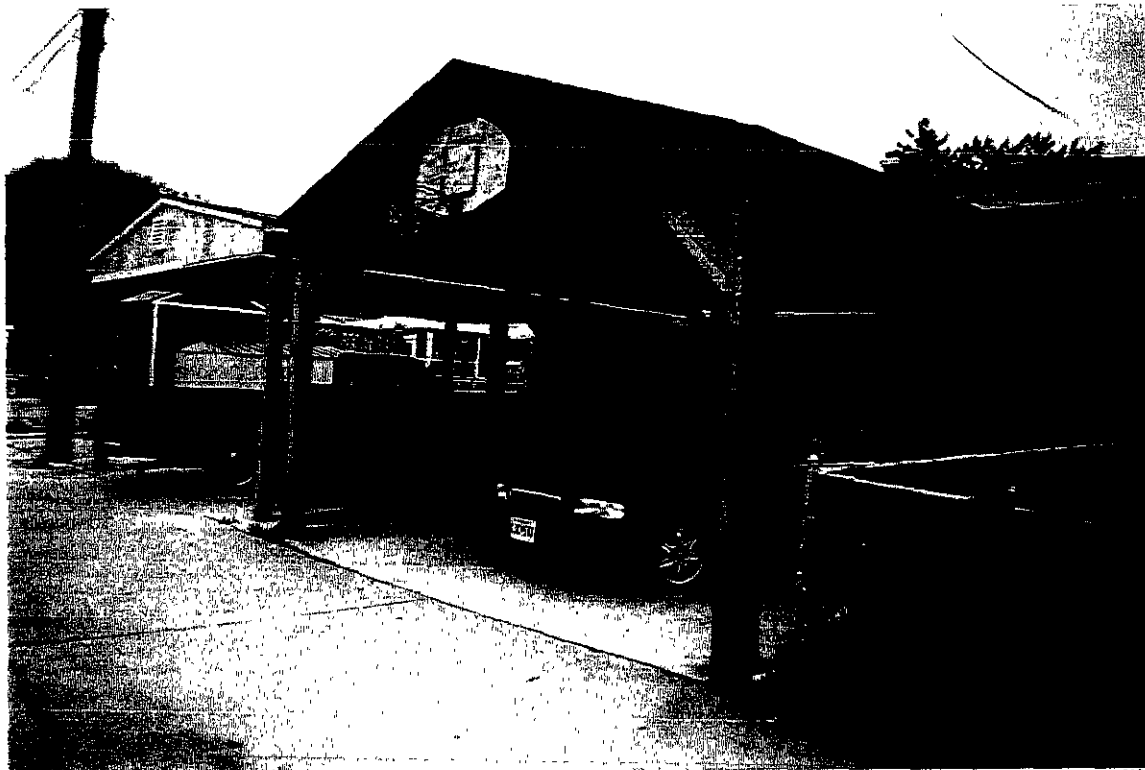
EAST SIDE OF CARPORT ↗
