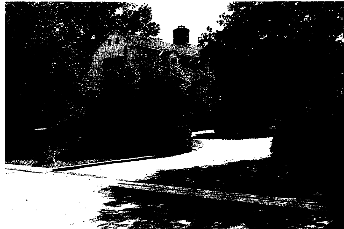
VIEW APPROACHING DRIVEWAY FROM WEST
