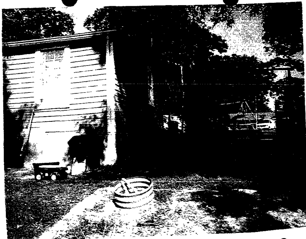
Standing on front yard looking at front East side of existing house.
