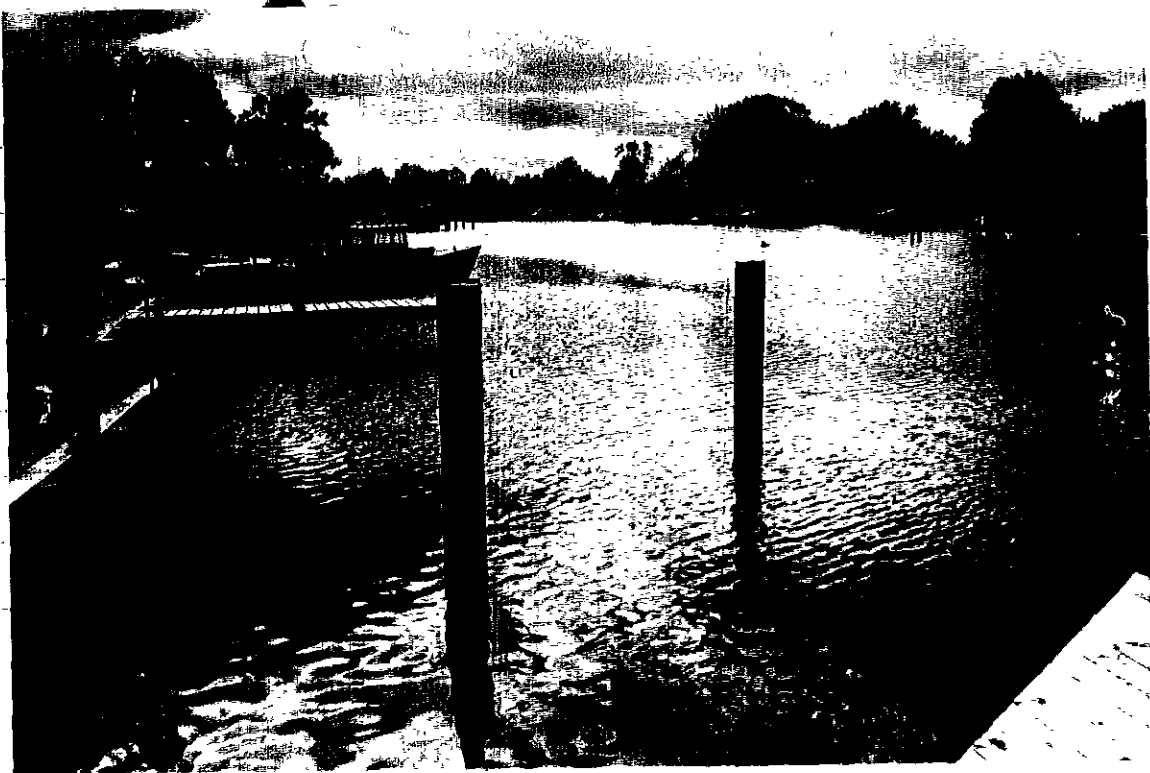
Pilings + neighbor's property
