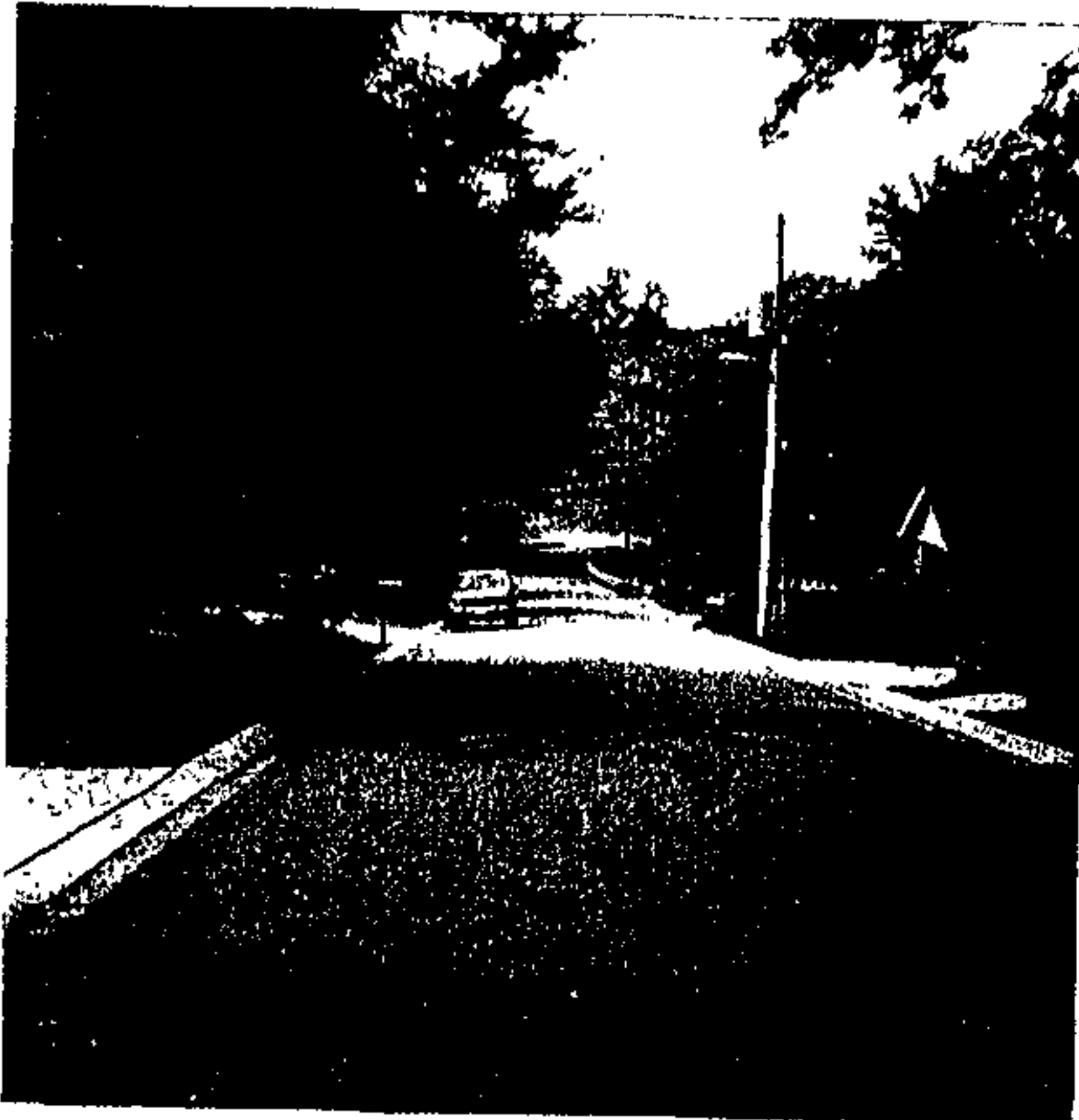
VIEW OF CATANNA AVE. 5. LOOKING WEST.
