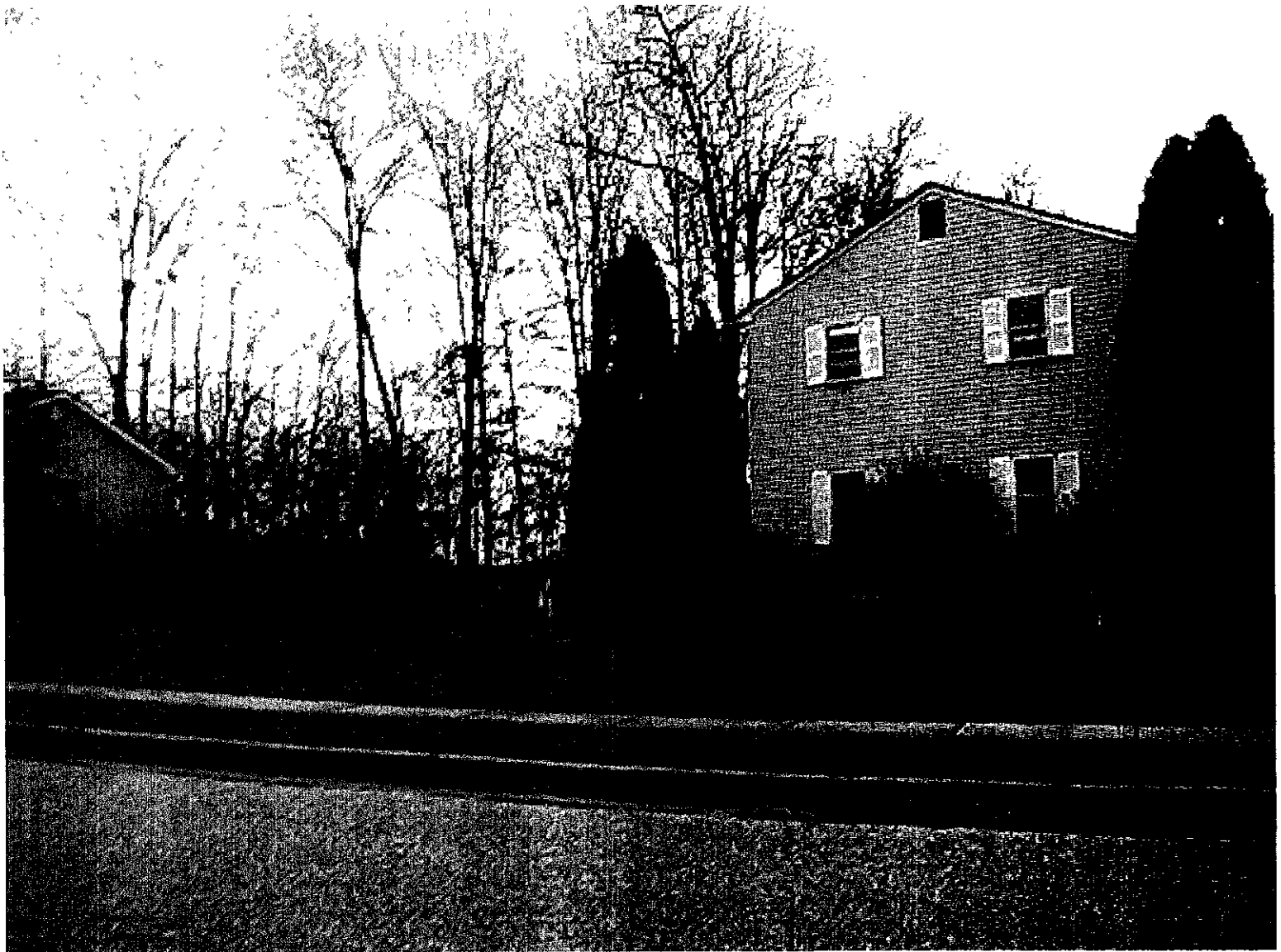
UNION HALL Ct. View from side street
