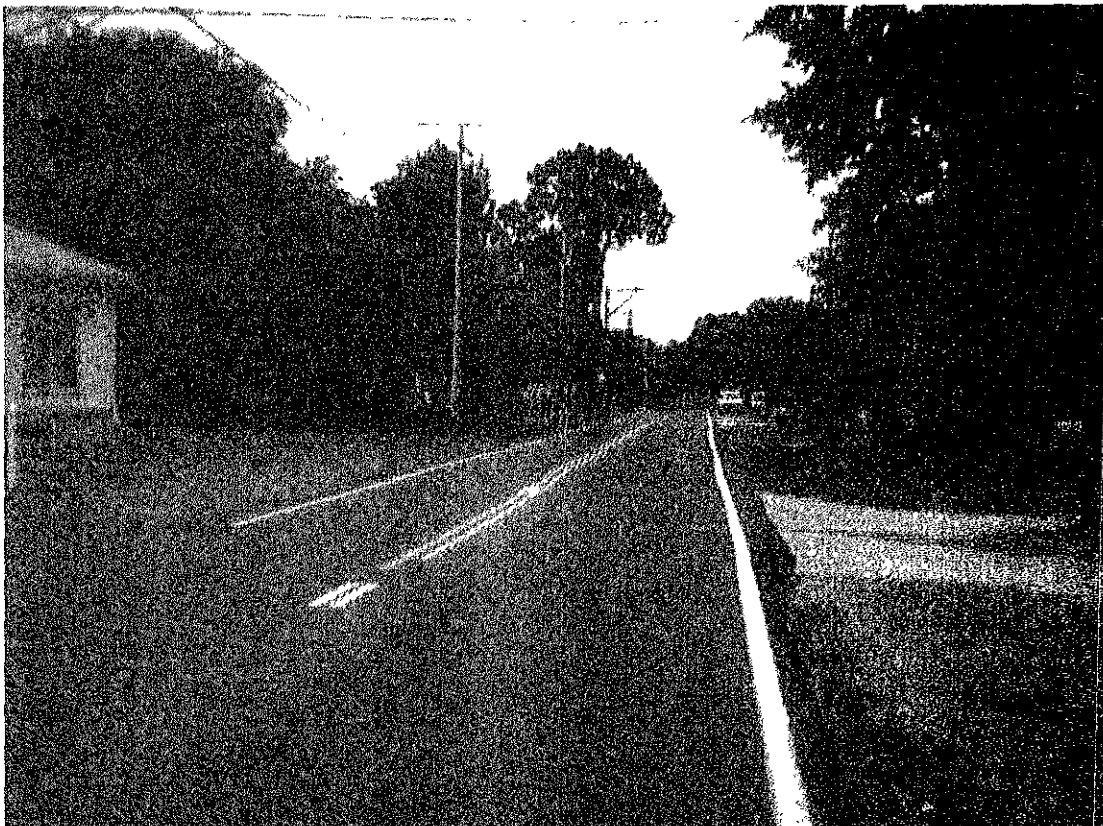
RIVERSIDE LOOKING SOUTH
