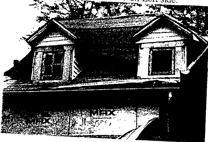
11. 104 McCormick Ave., Fire damage.
