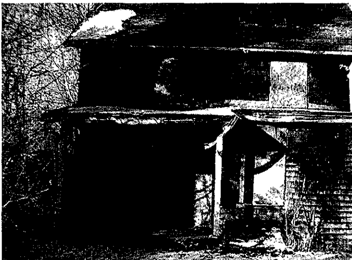
Back porch, collapsing.
