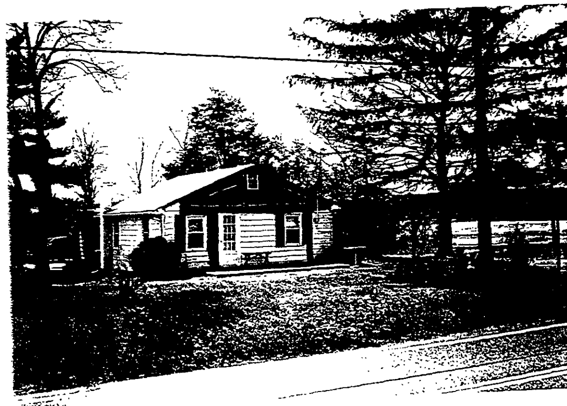
MIDDLETOWN ROAD VIEW OF PORCH REMOVED
