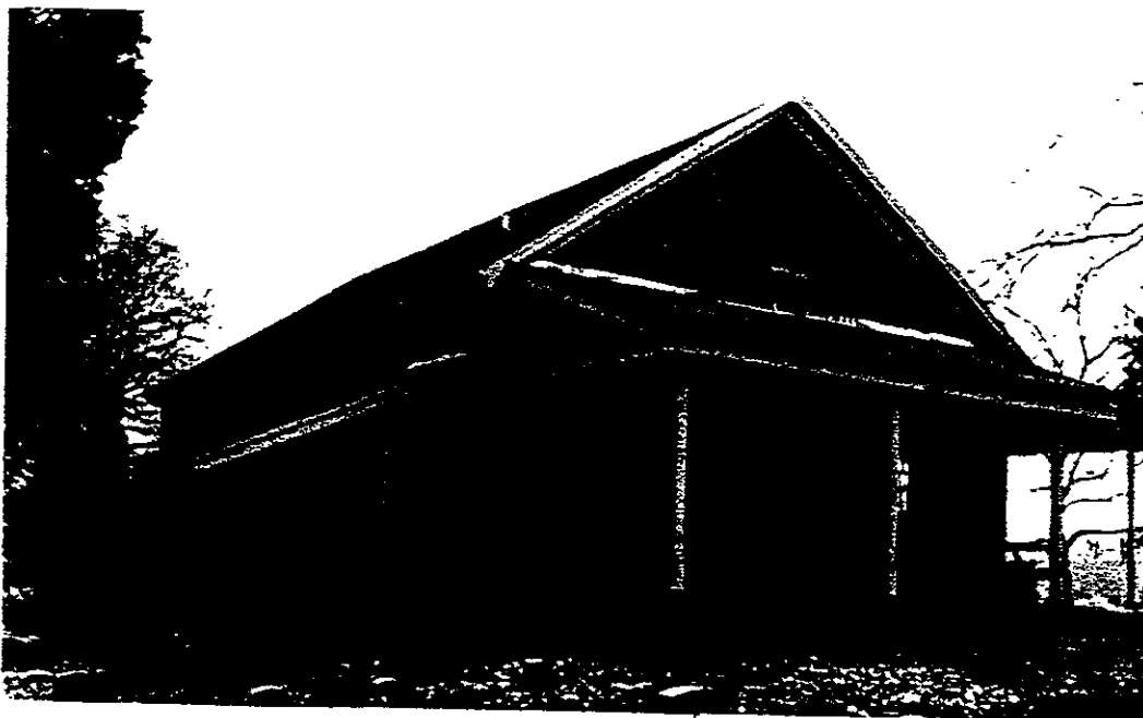
Existing rear and side view of Meeting House
