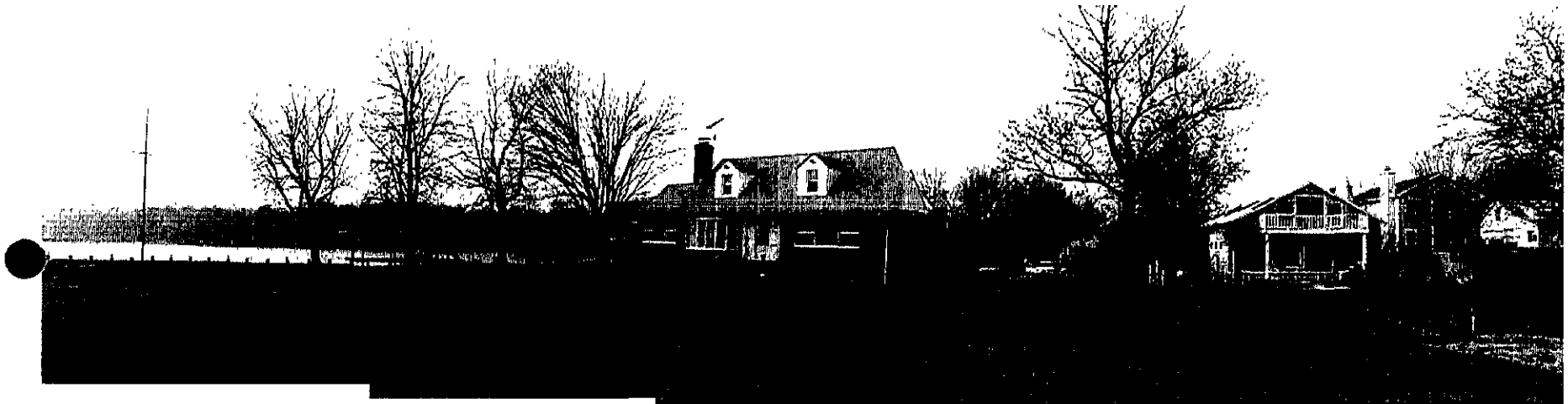
VIEW WEST OF EXISTING 3 HOUSE FROM WATER
