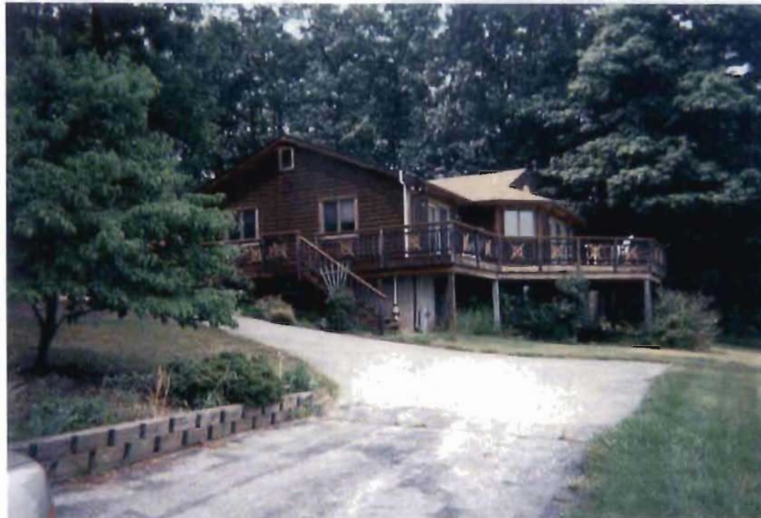
5. South elevation #21444 Dunk Freeland Road.
