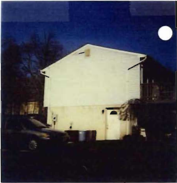
#500 Proposed side of house where addition would be located
