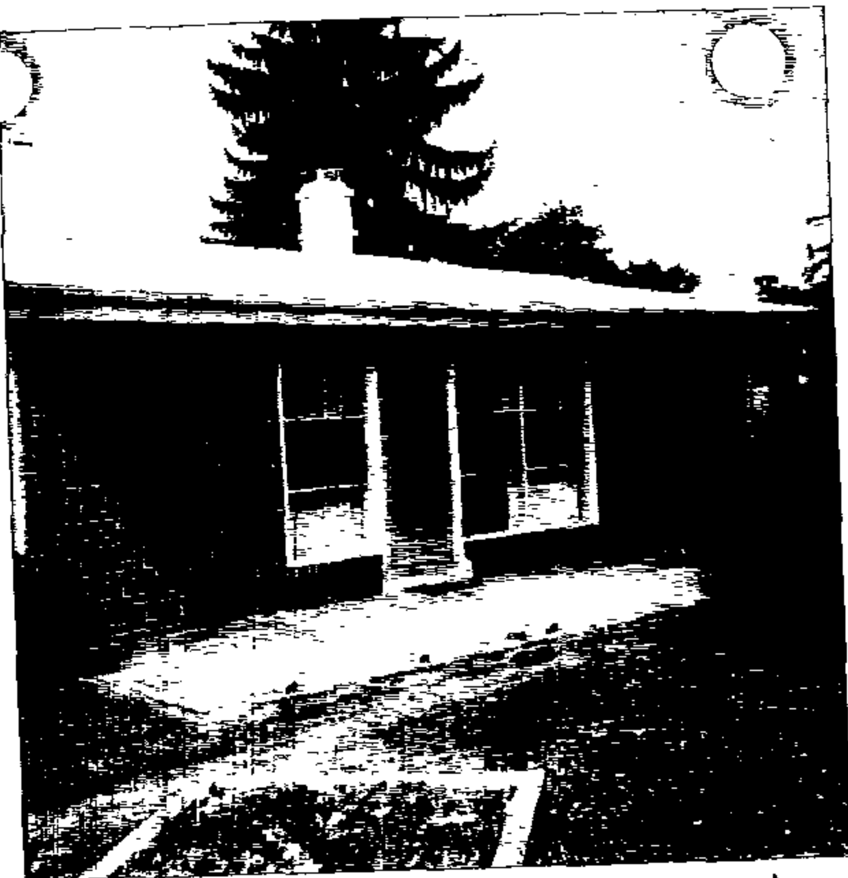
Left side of #27 7414 Kalton Ct
