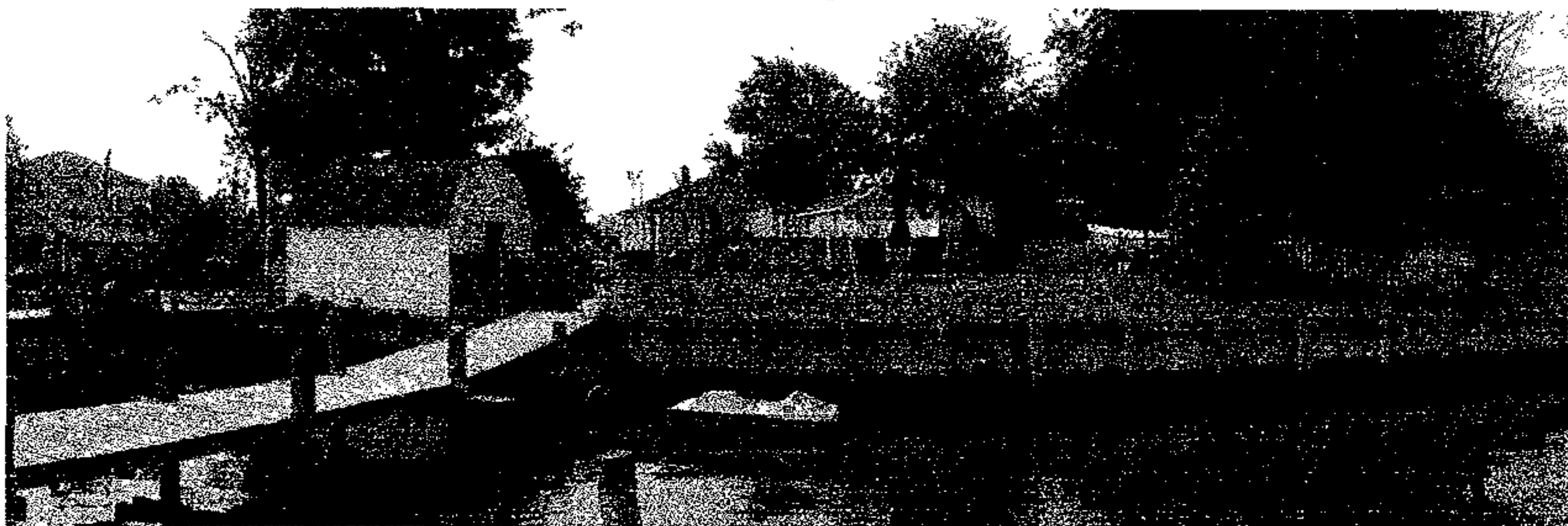
REAR OF PROPERTY FROM PIER
