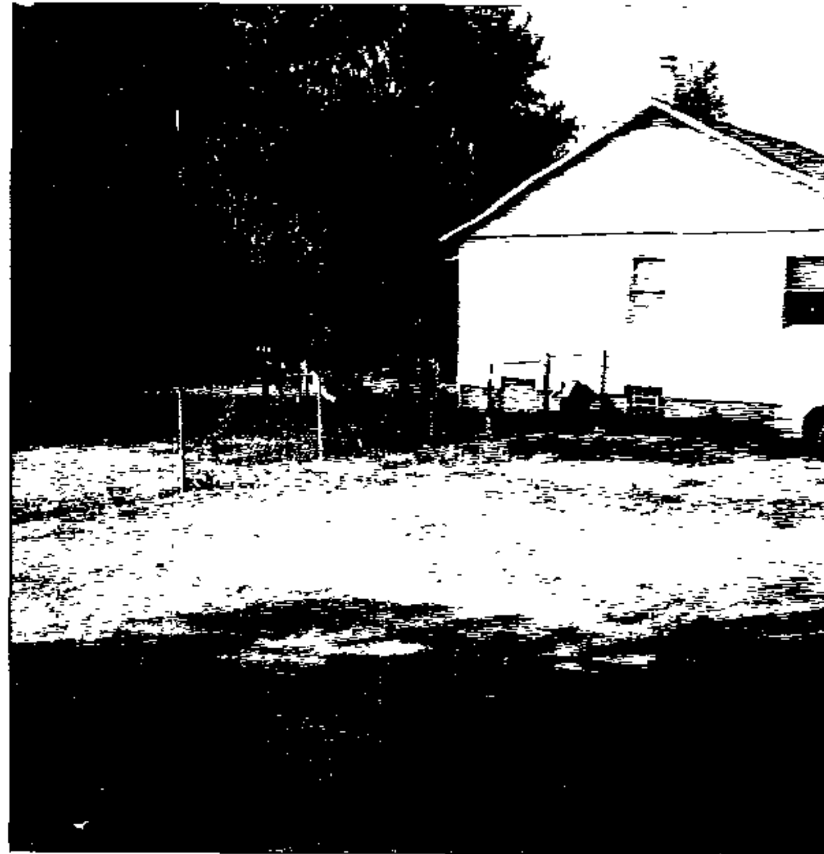
SIDE VIEW-2 #9 OF BLDG. SITE
