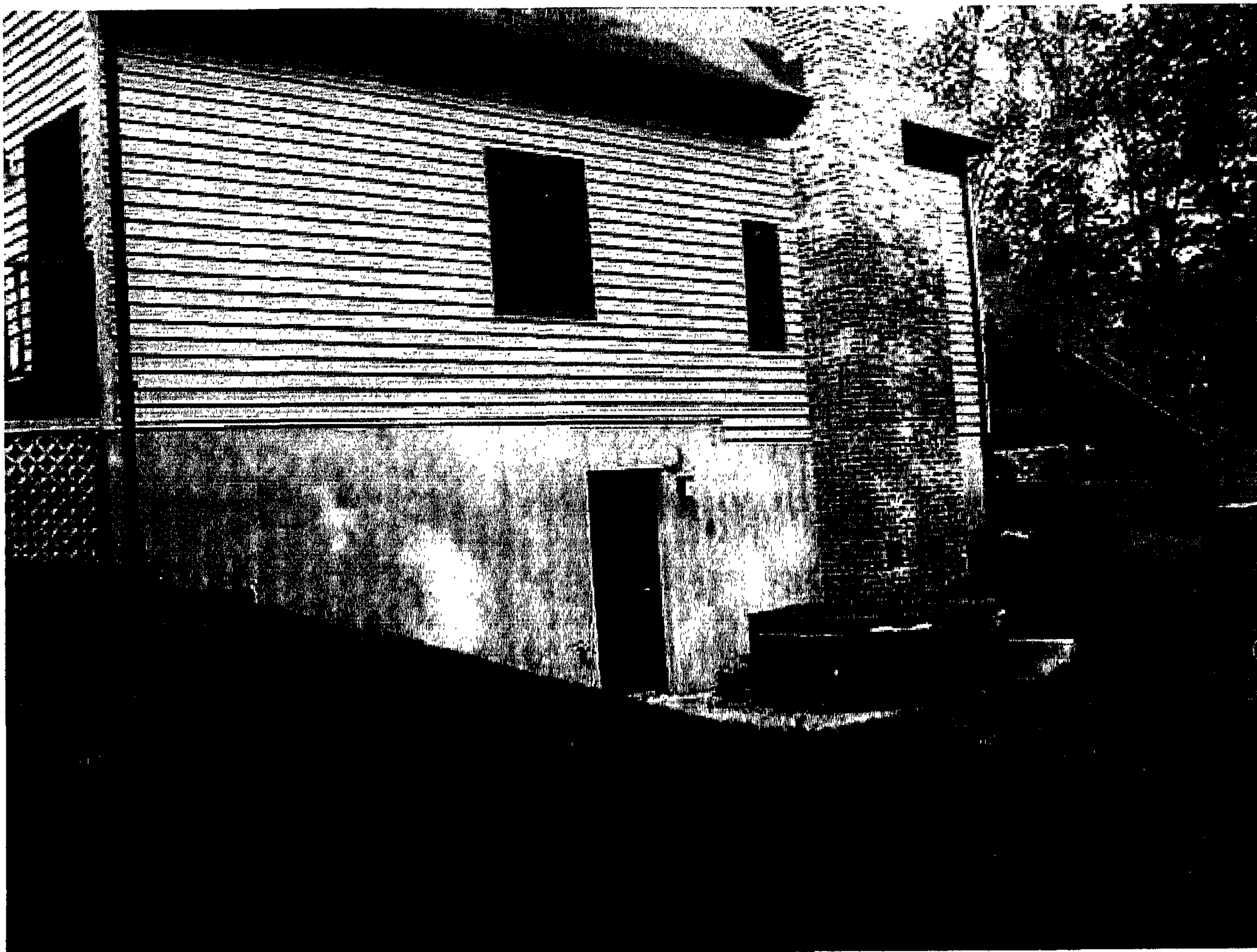
Side of house 10207 Plettenberg Rd
