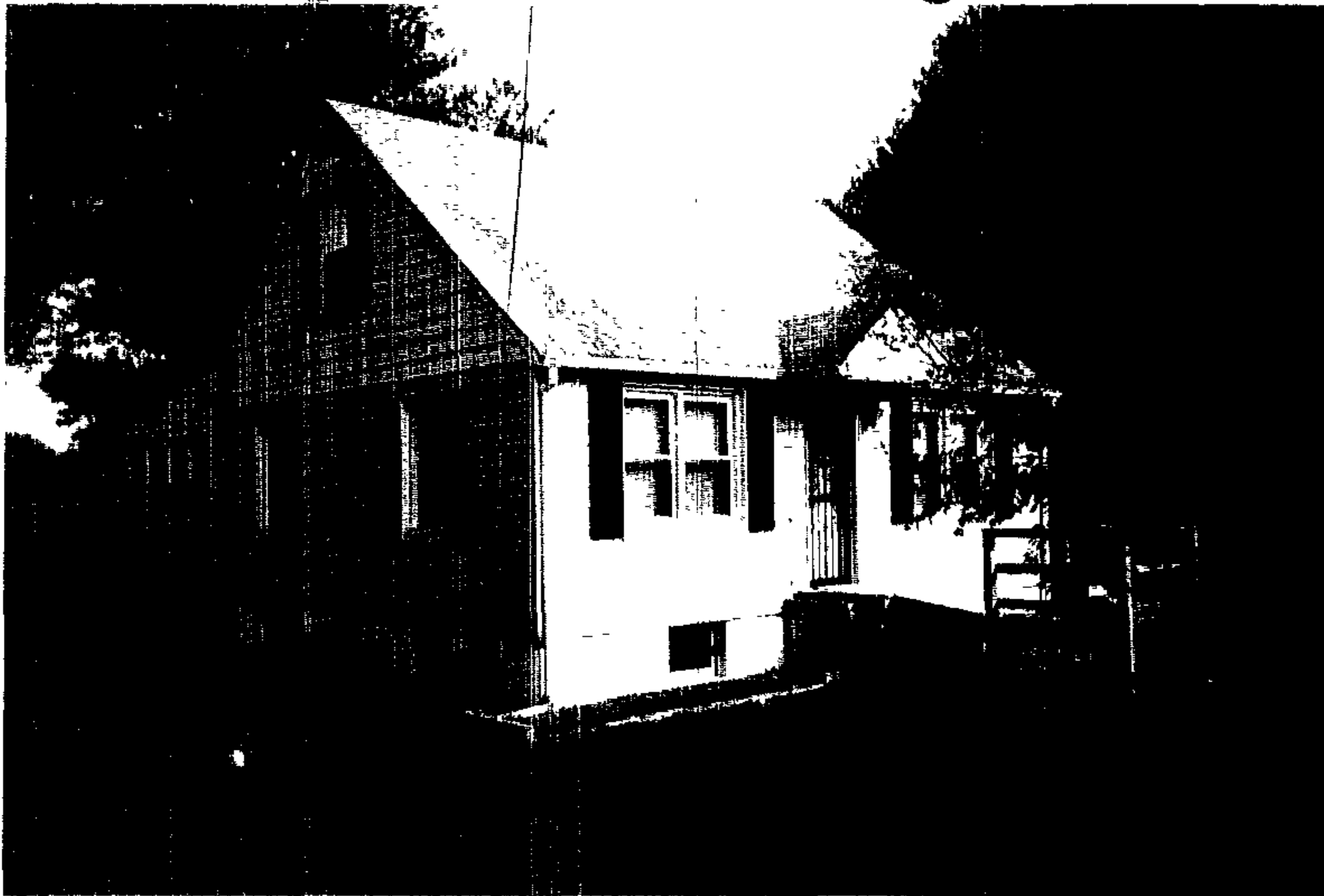
FRONT OF HOUSE SHOWING NORTHWEST CORNER – LOCATION OF PROPOSED 8' X 12' ADDITION
