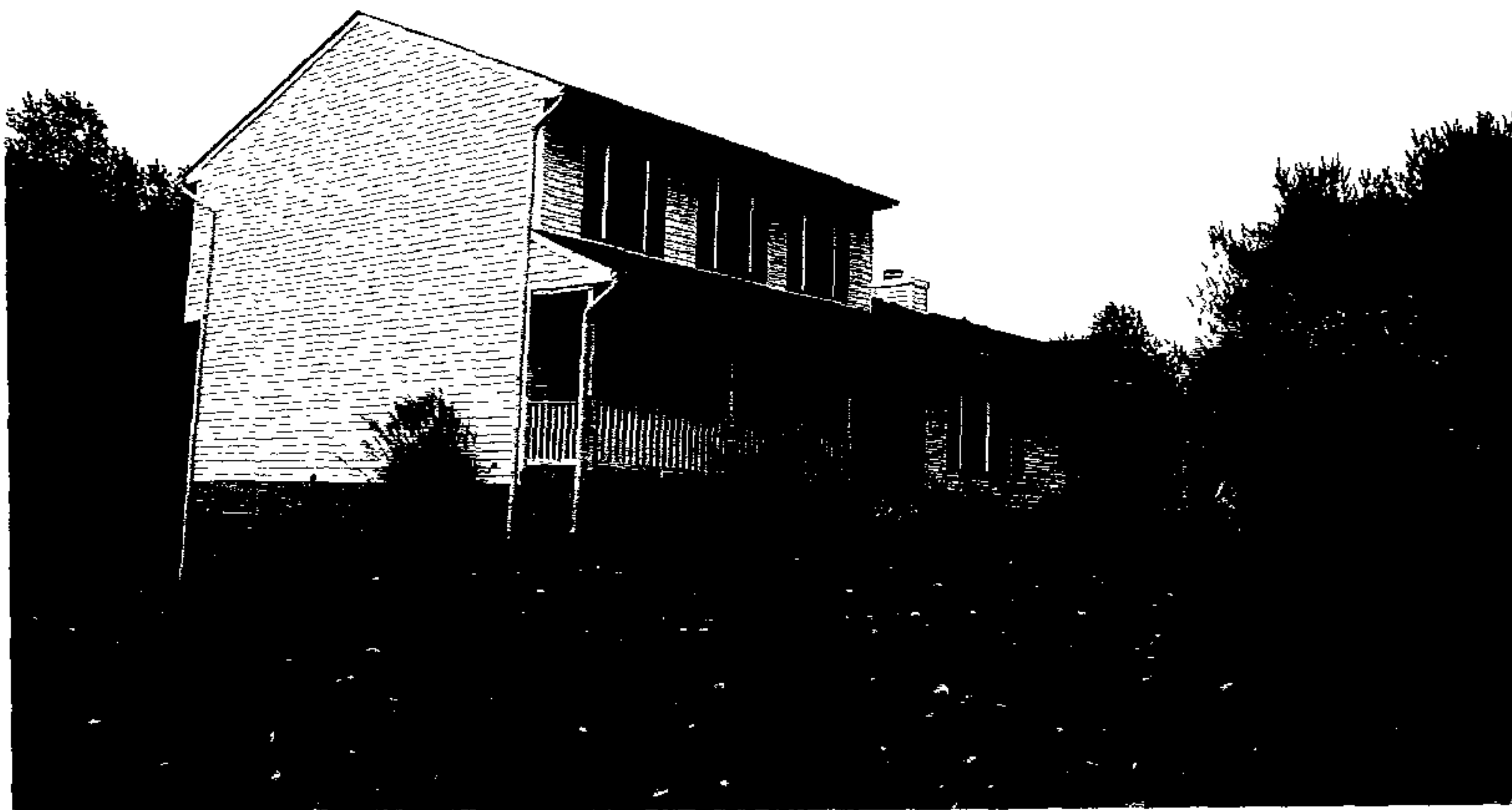
Photo 5. Addition will be built on left side of house
