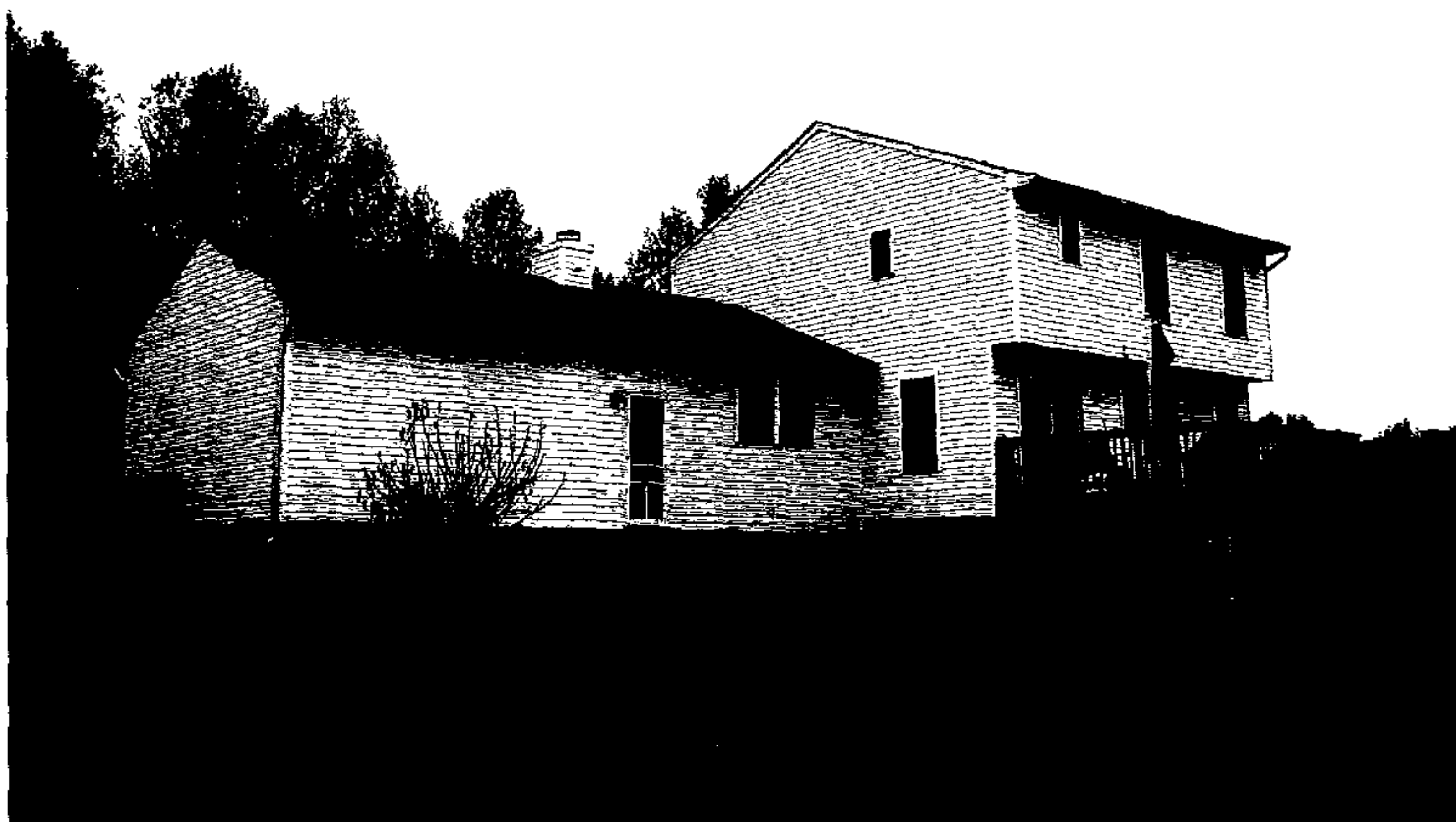
Photo 4- Rear of house showing garage.
