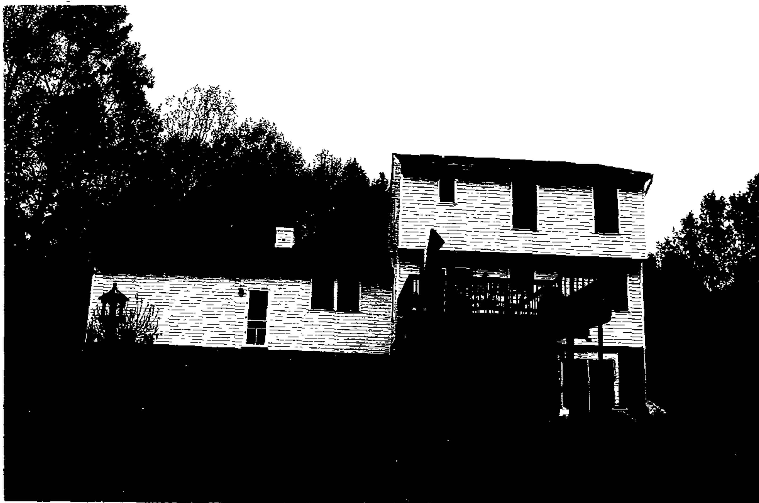
Photo 2 - Rear view of house. Addition to be built on Right of house
