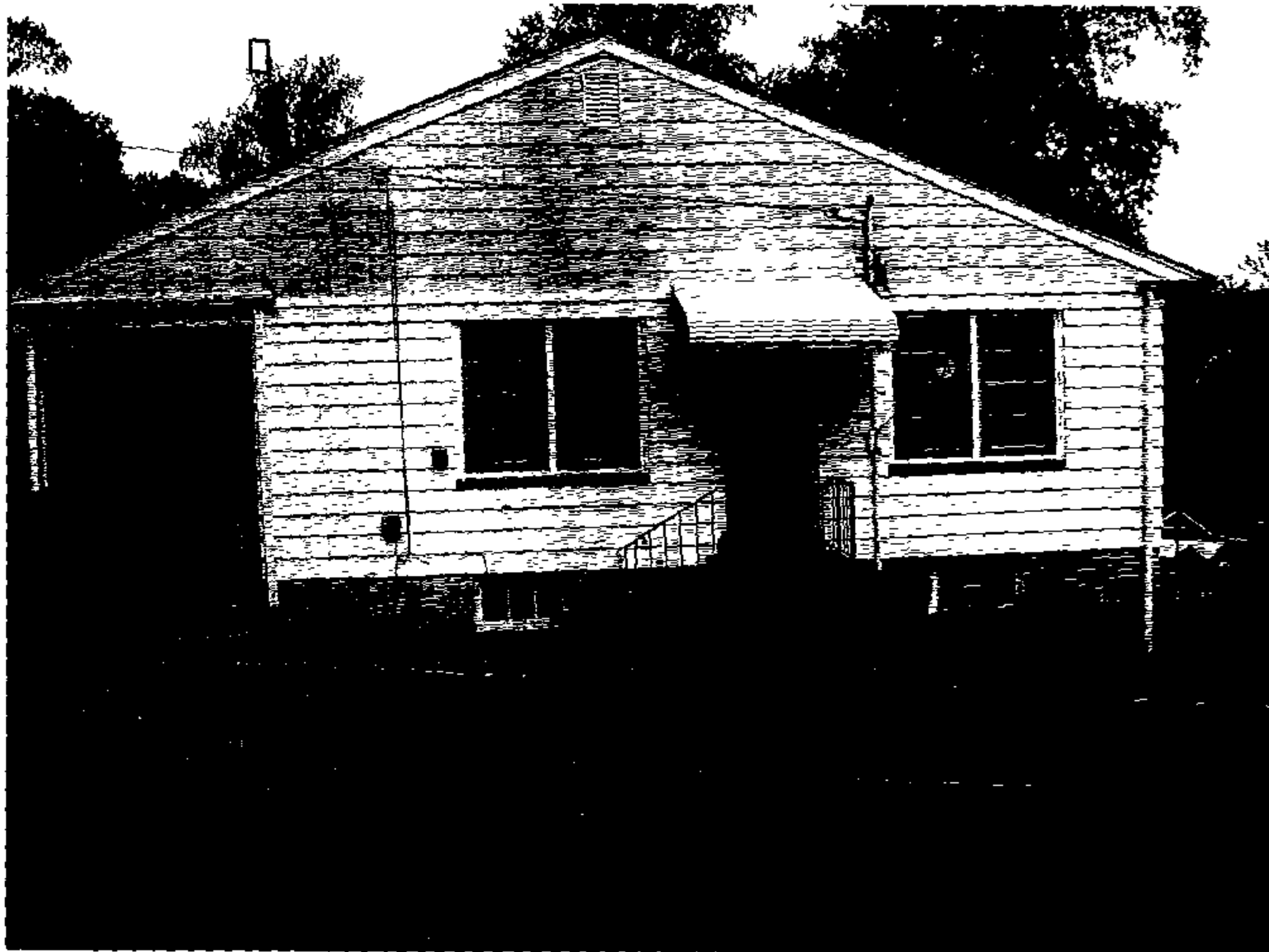
View of 511 Hilton Ave from southern neighbor (515 Hilton Ave)
