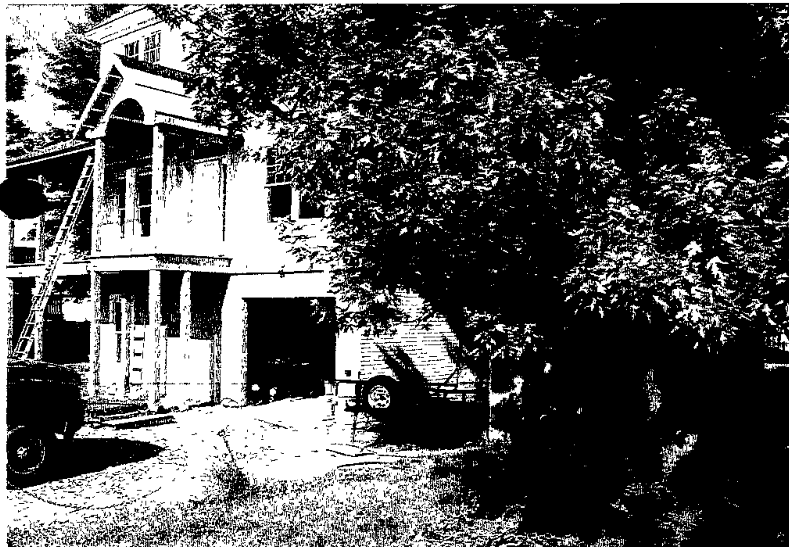
VIEW TO LEFT FROM EXISTING
