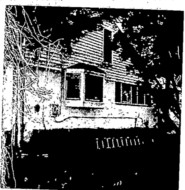
front left right side of house
