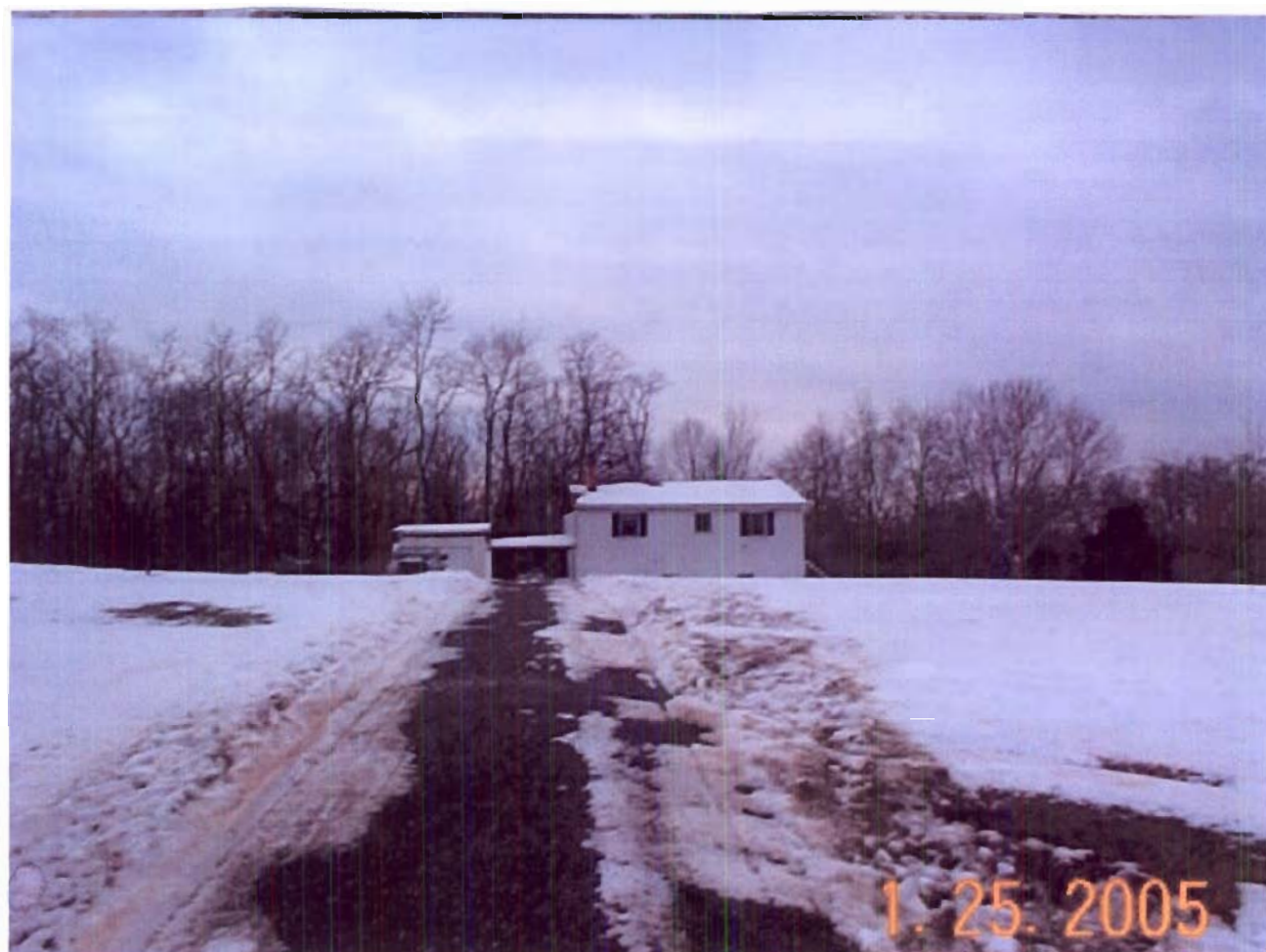
From Piney Grove Rd - driveway leads to dwelling - Pole structure is between Piney Grove & dwelling.
