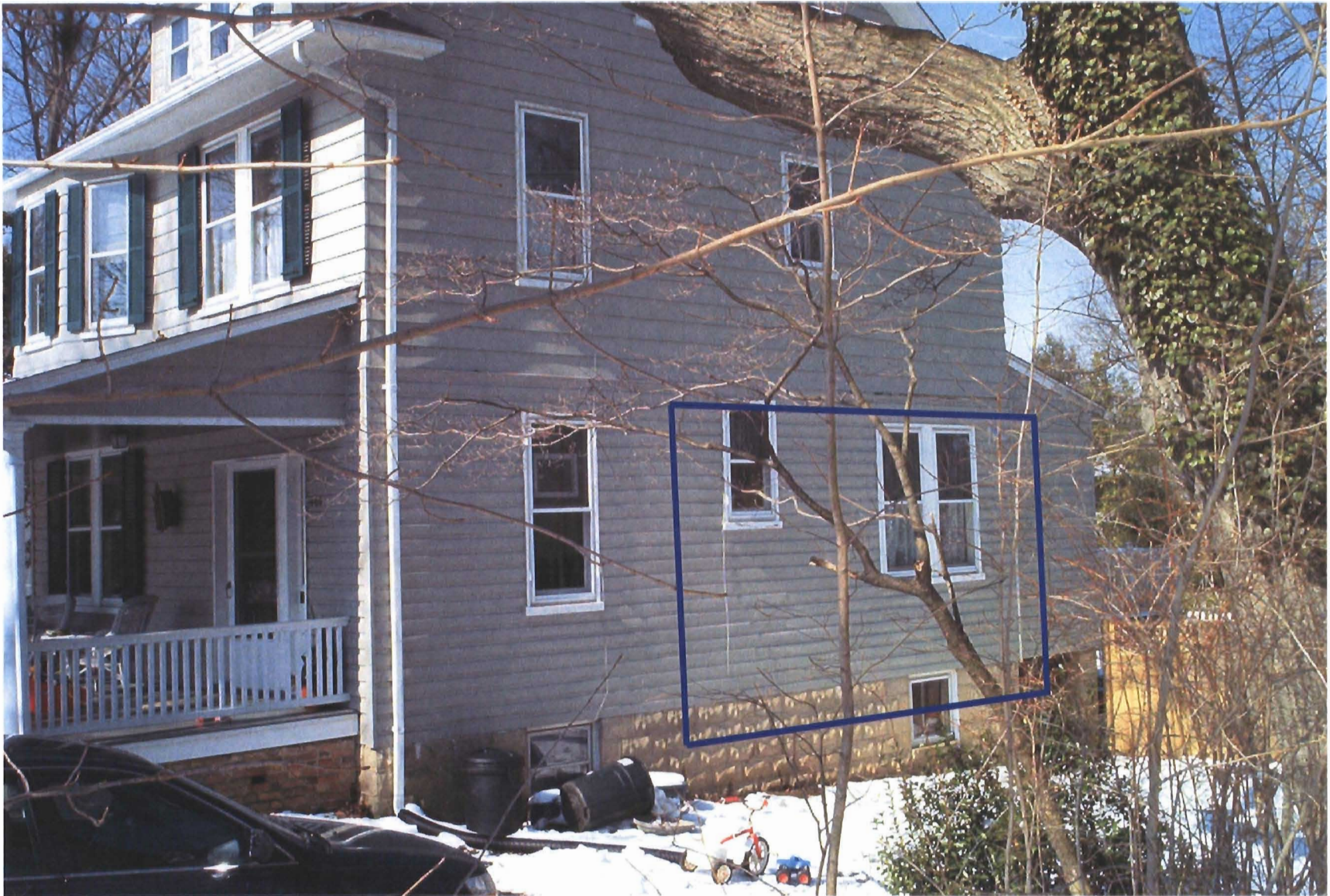
This photo shows the area of the east side of 1404 Summit where the proposed addition would be sited
