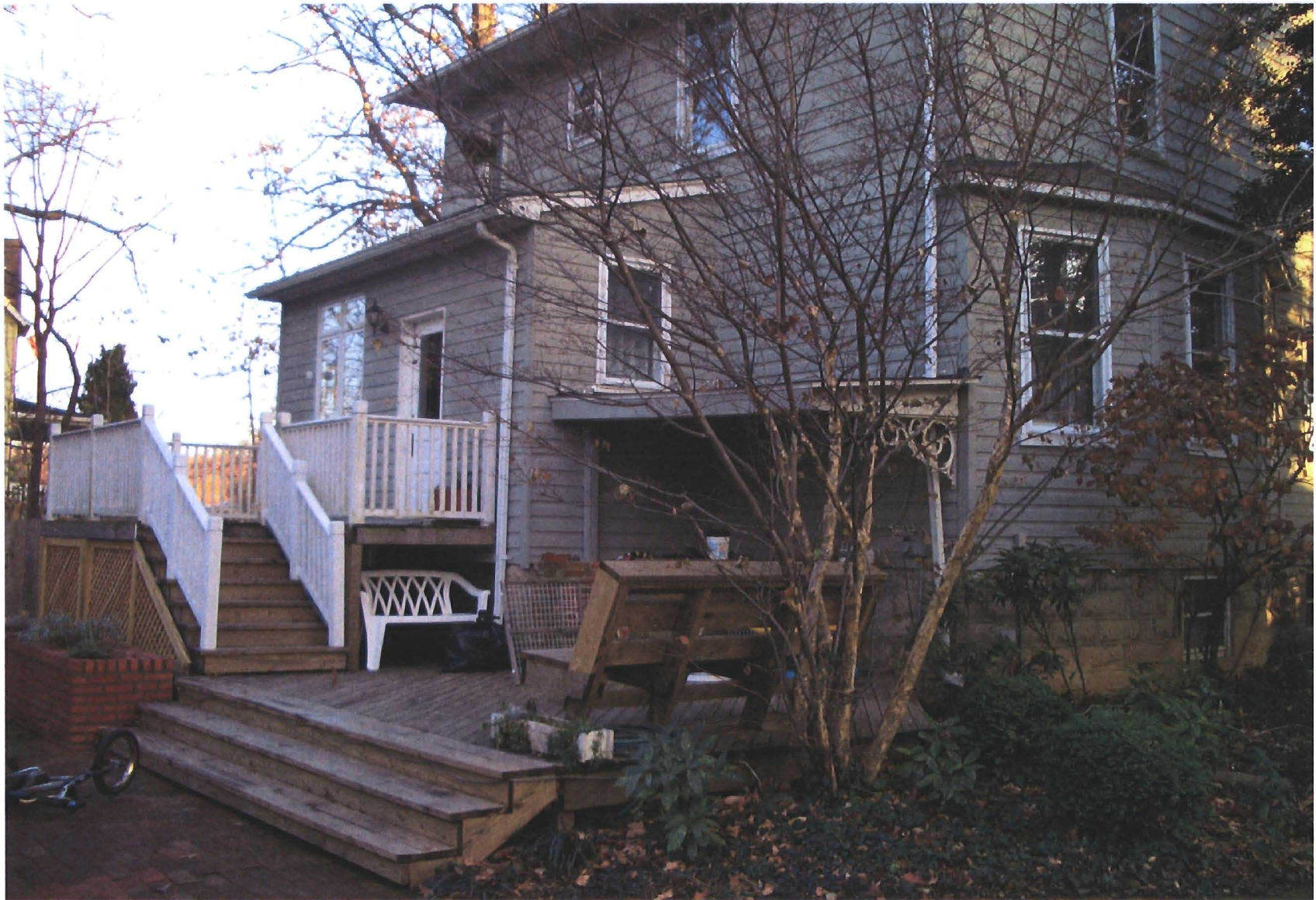
Back of house (view from northwest)
