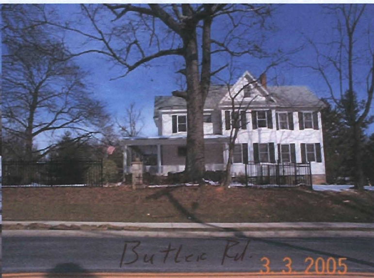
AREA OF Fence in Violation of Pool Enclosure Requirements
