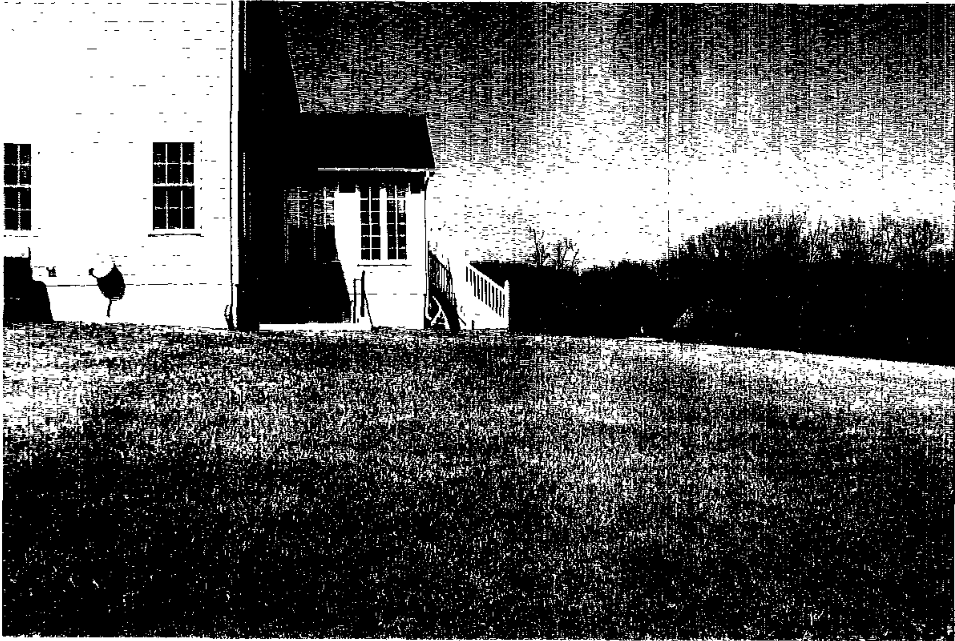
SOUTH SIDE OF HOUSE LOOKING NORTH AT PROPOSED SITE
