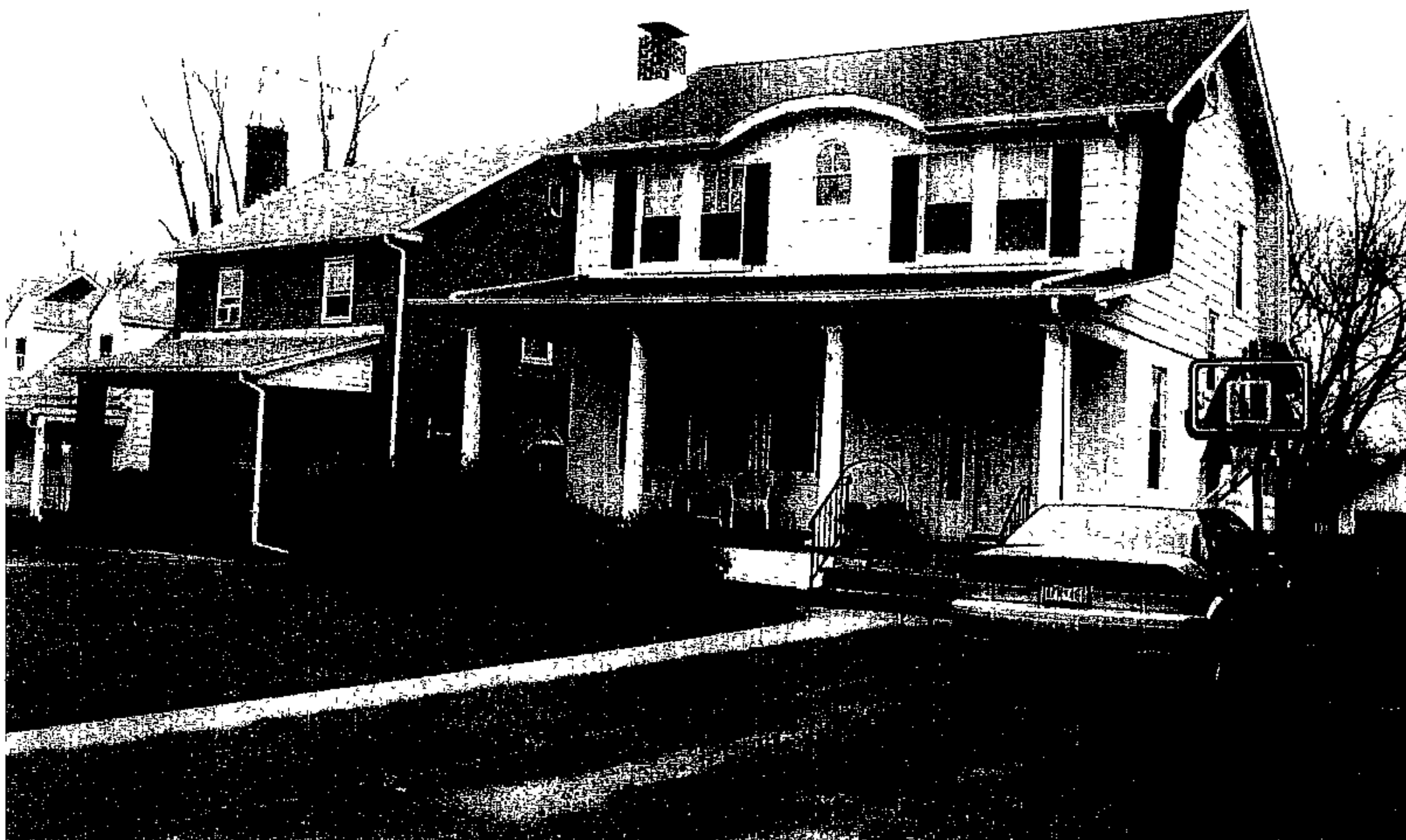
FRONT OF PROPERTY AND ADJACENT PROPERTY ON EAST SIDE
