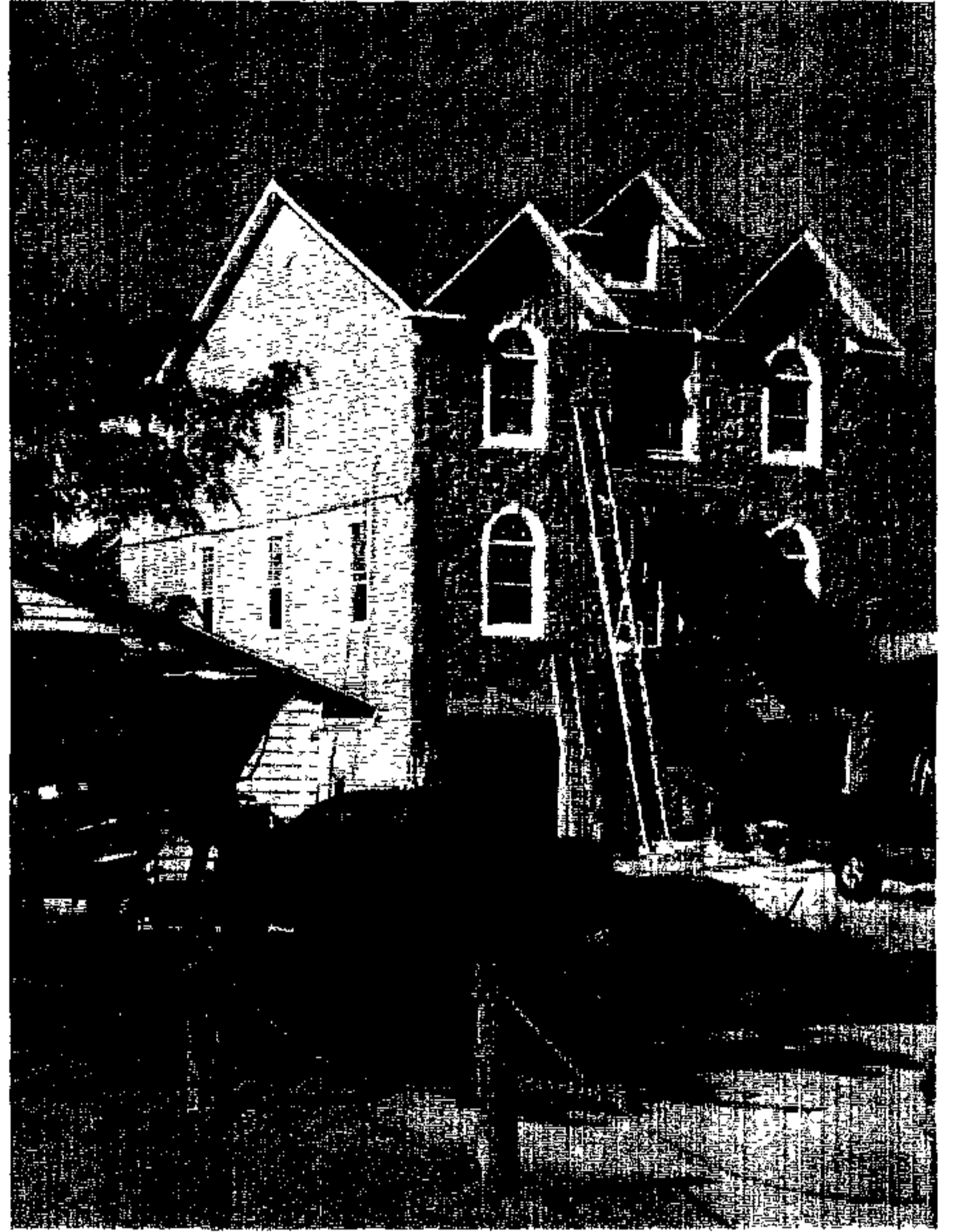
1226 Burke Road (45 feet)
