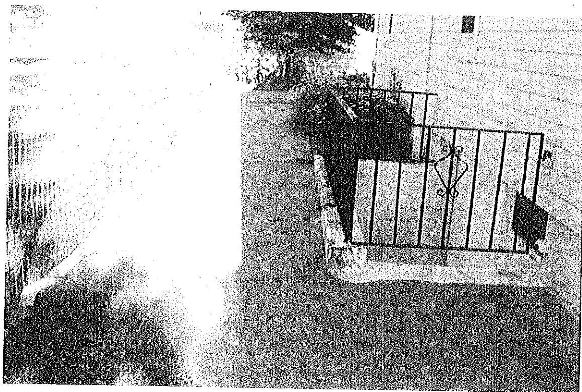
View from Side of house
