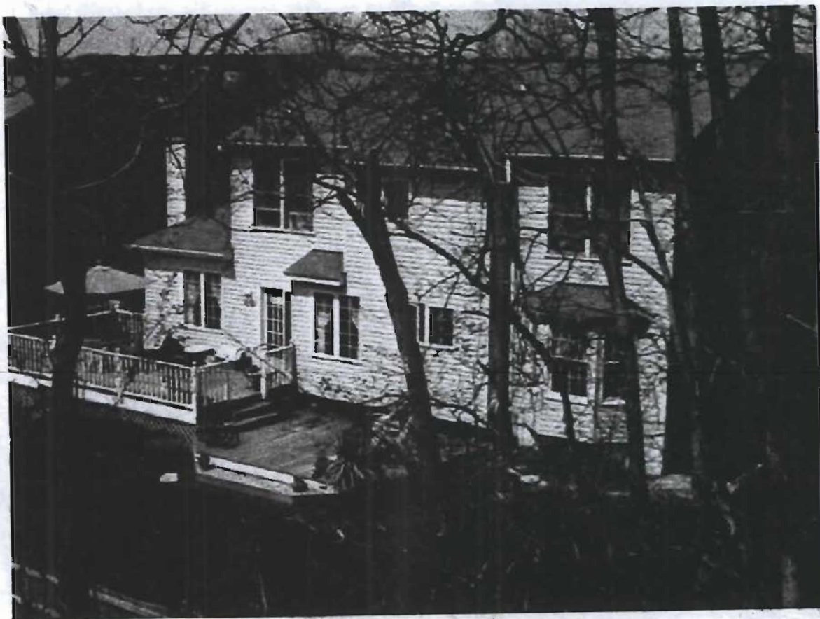
→ Back of House. Deck in which to be built opp
