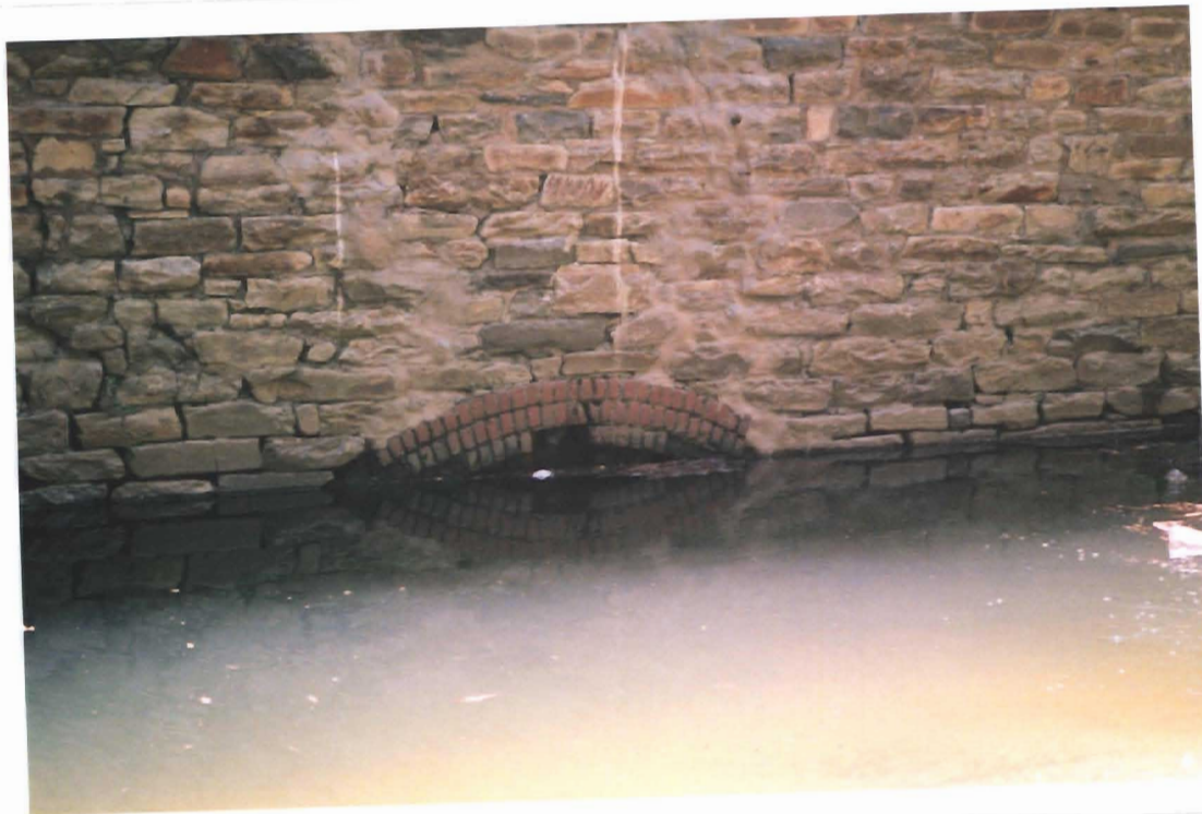
PHOTO 6: CULVERT, BACKUP TOWSON RUN INTO LAKE ROLAND
