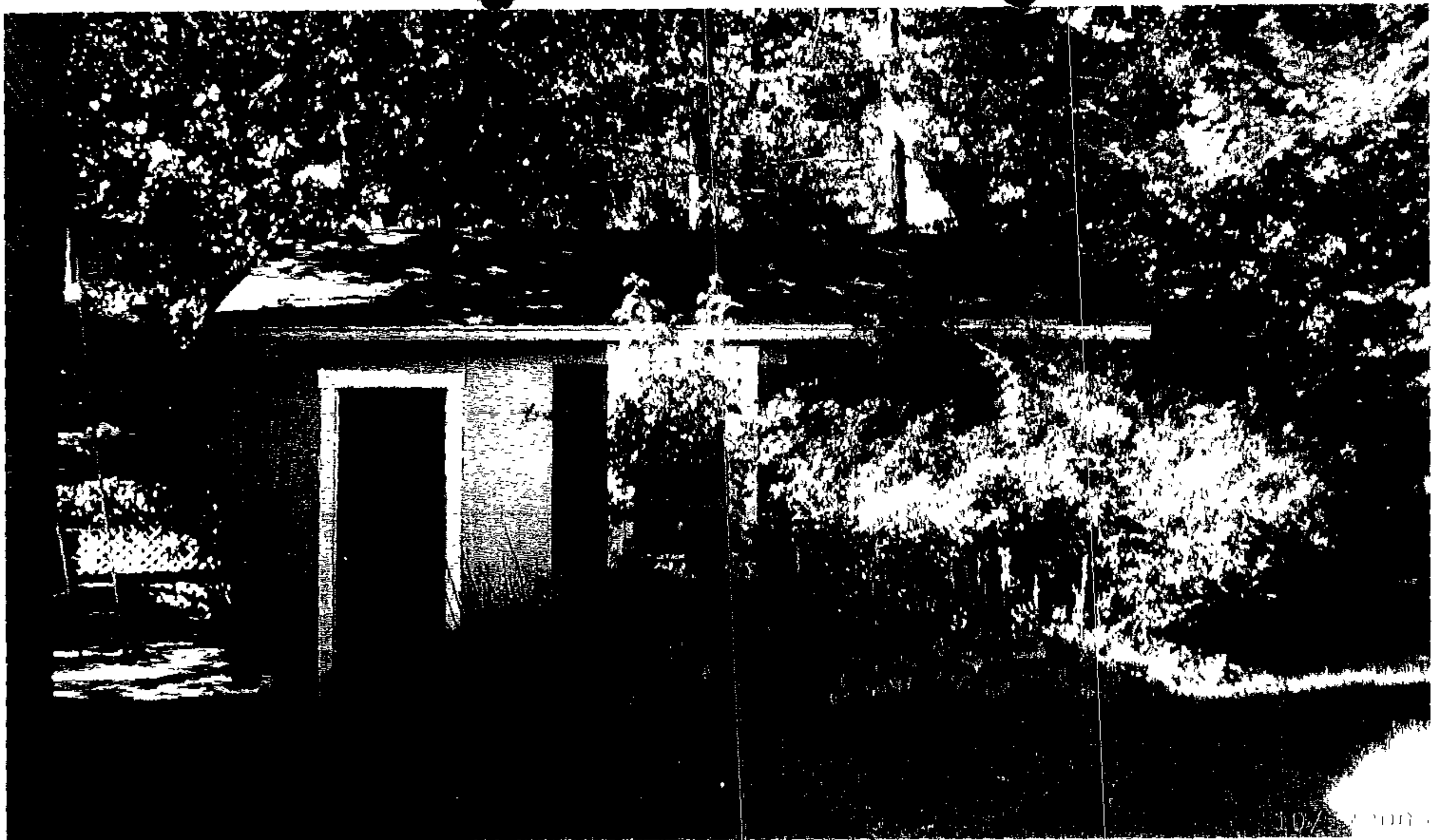
East elevation of Garage
