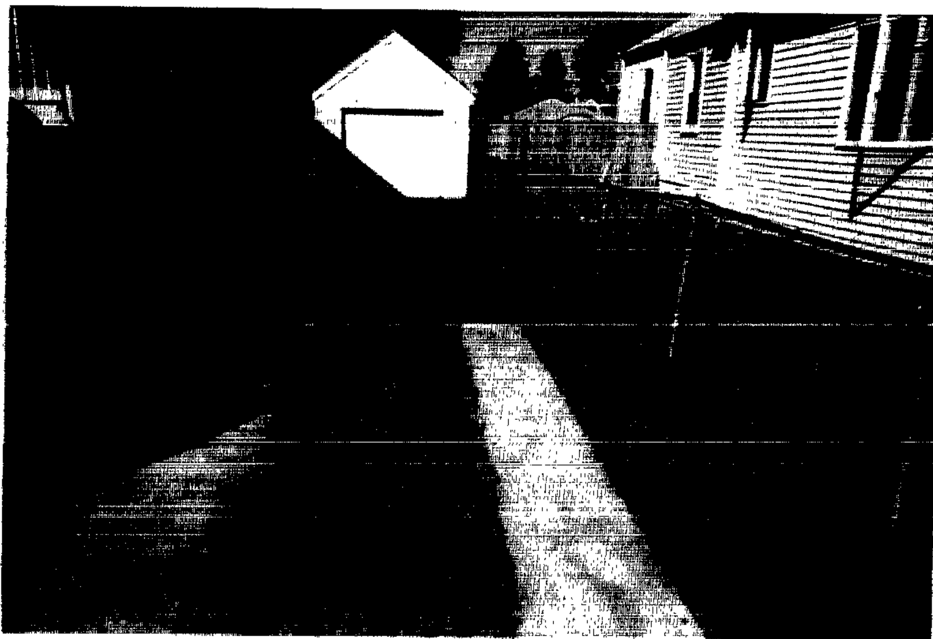
OLD GARAGE TO BE TORN DOWN DUE TO AGE AND CONDITION
