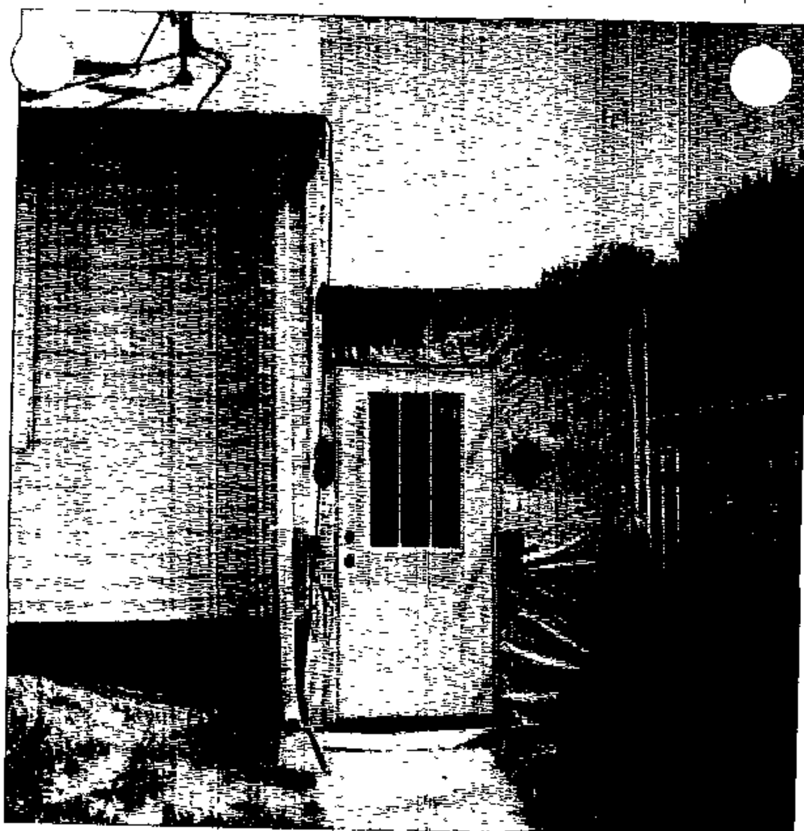
View of door to Basement 3E steps. From Back Yard. OG-659-A
