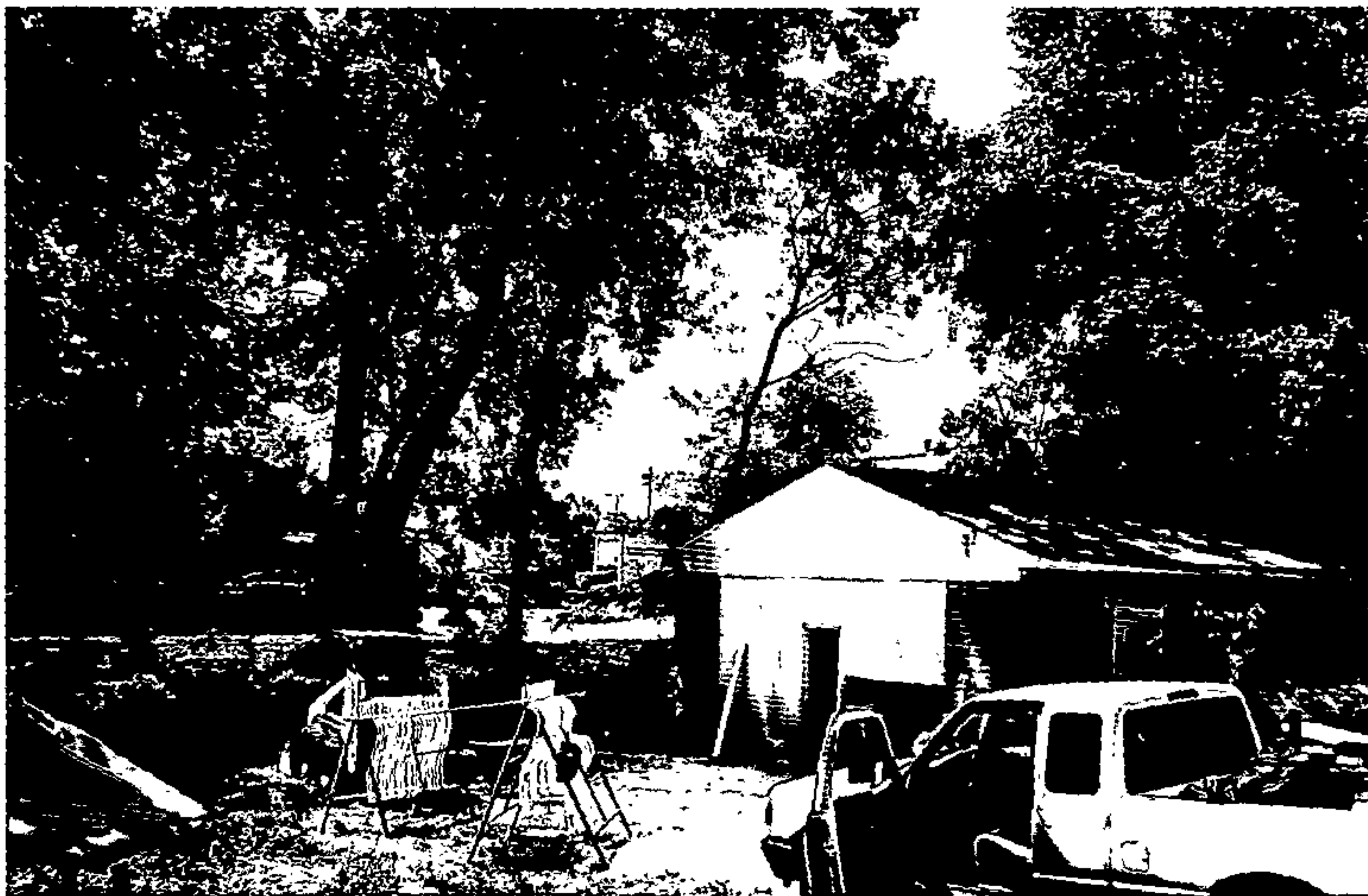
View of existing garage toward truck parking lot.
