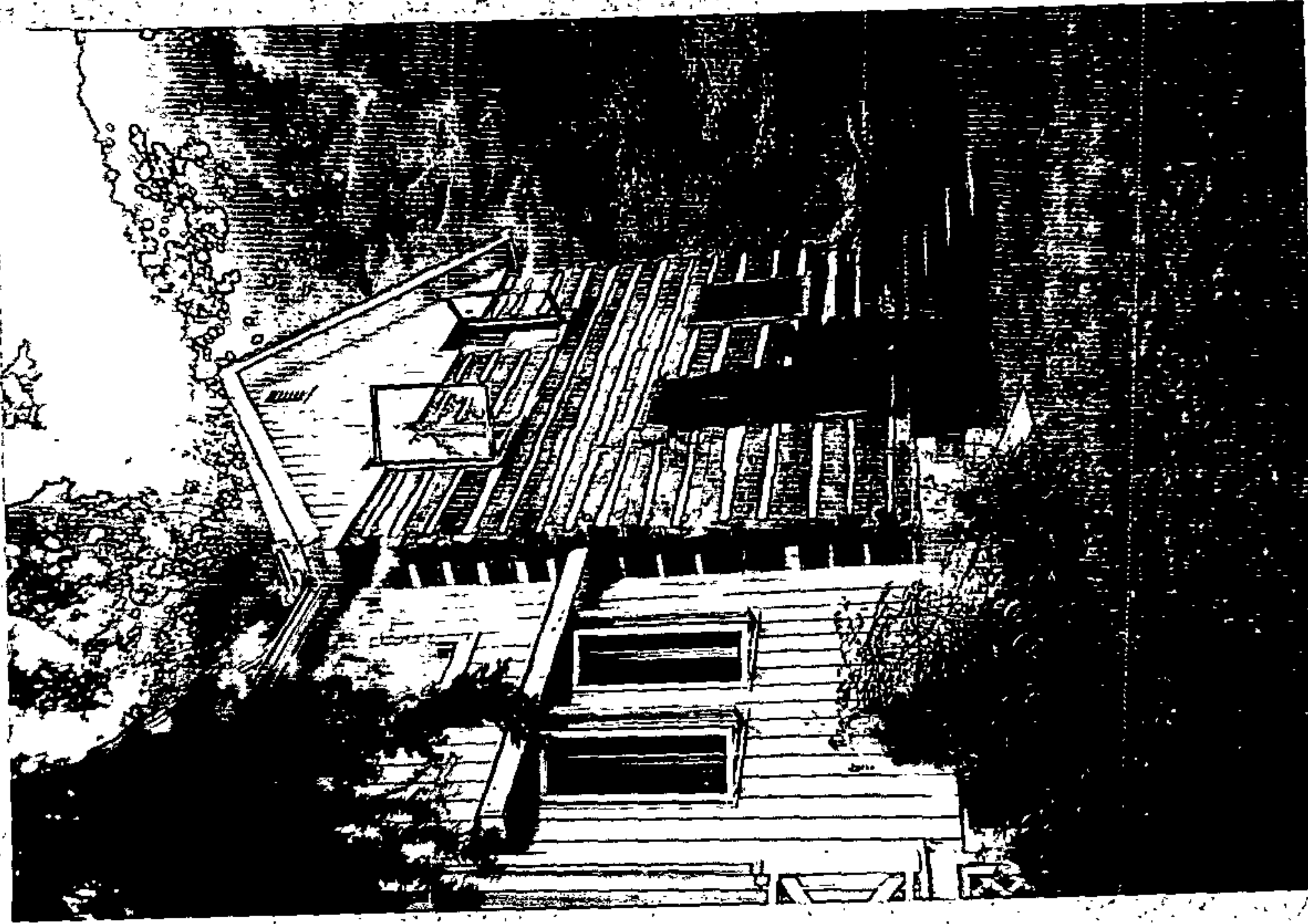
19. S. FACADE OF 10707 SHOWING FULL DOVE TAIL CORNERS.
