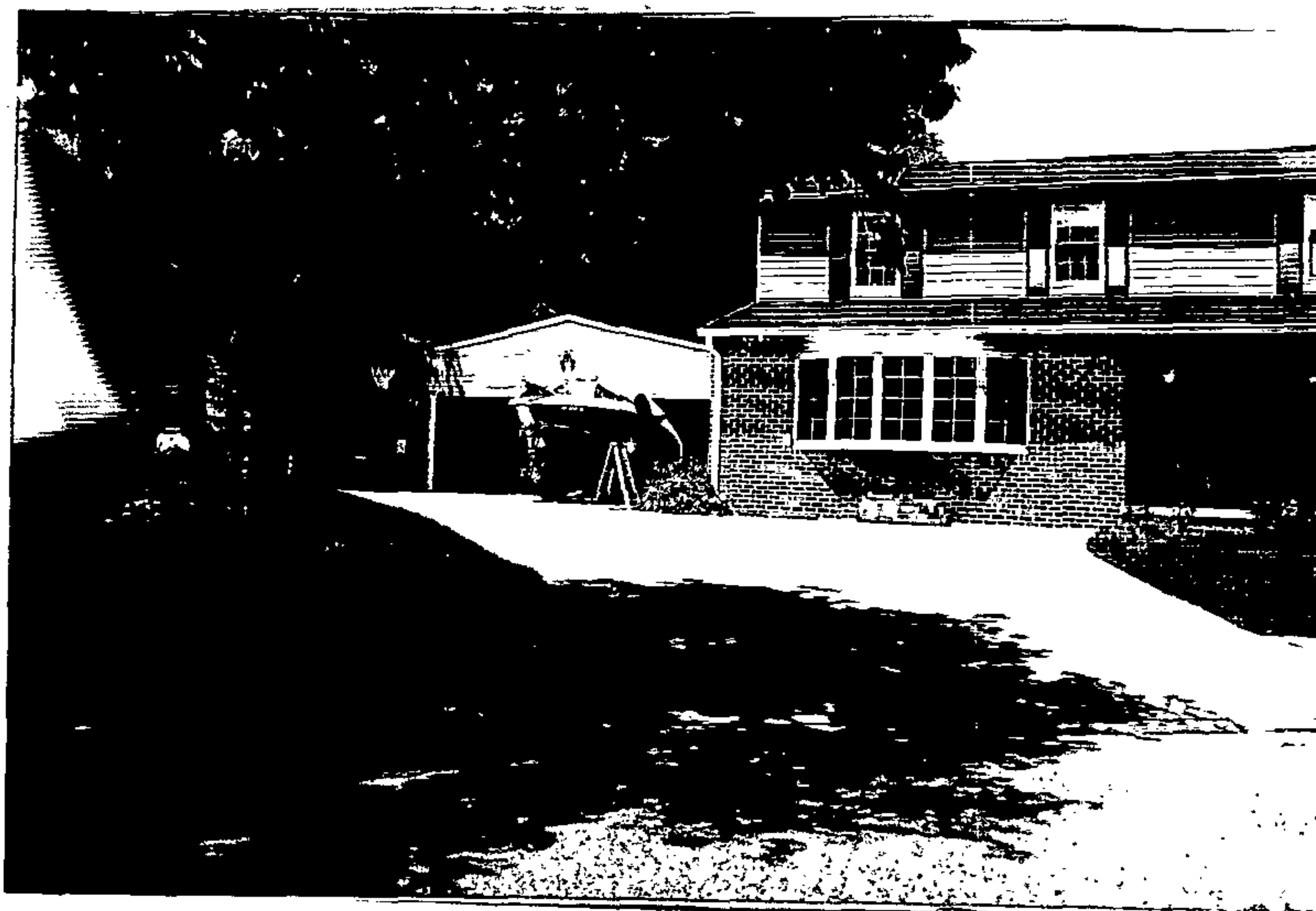
20. 10708 Added a full two-car garage side of the house, bumped out a window from the old garage that was turned into a family room.
