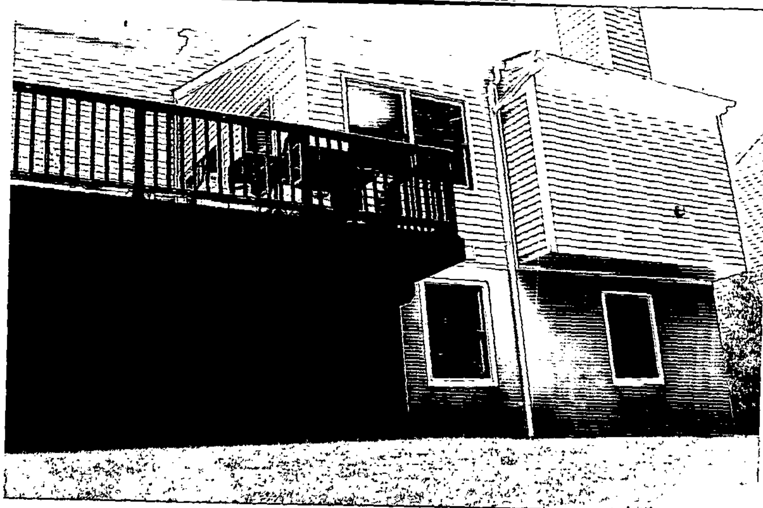
6. 10623 two-story Addition- view from the easement
