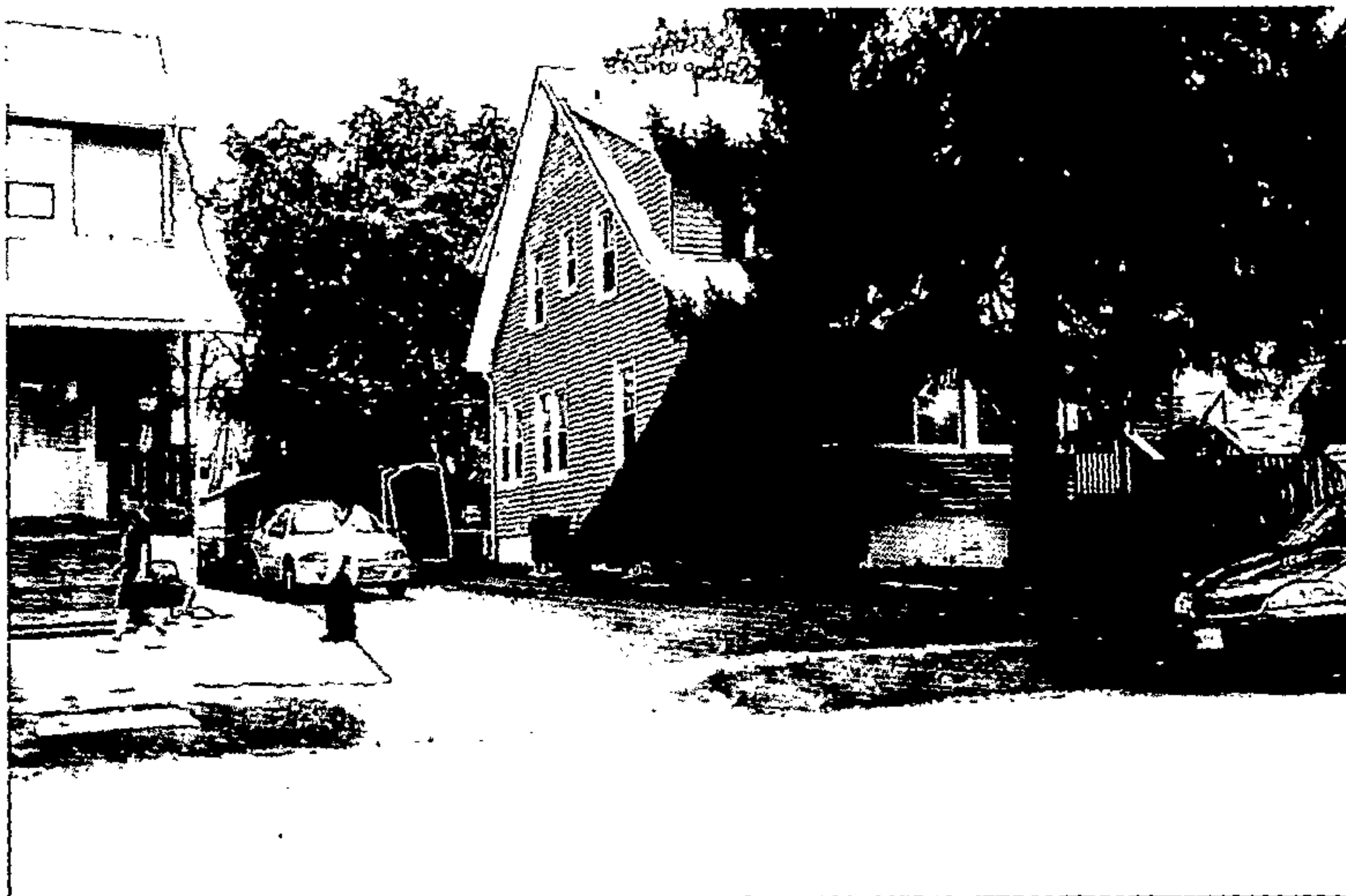
SOUTH SIDE AND FRONT VIEW OF 5548 CARVILLE AVENUE (5550 CARVILLE AVENUE TO THE LEFT OF PHOTO)
