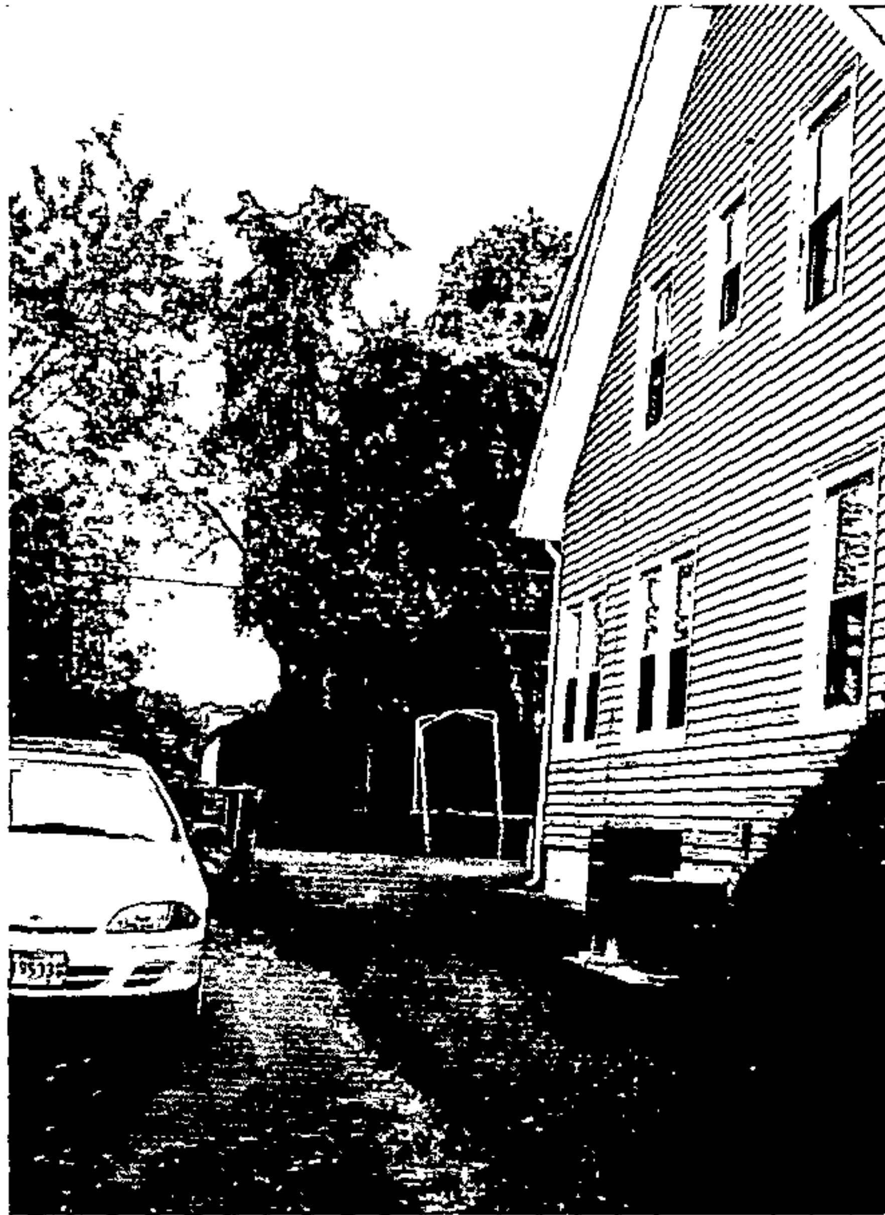
SOUTH SIDE OF 5548 CARVILLE AVENUE
