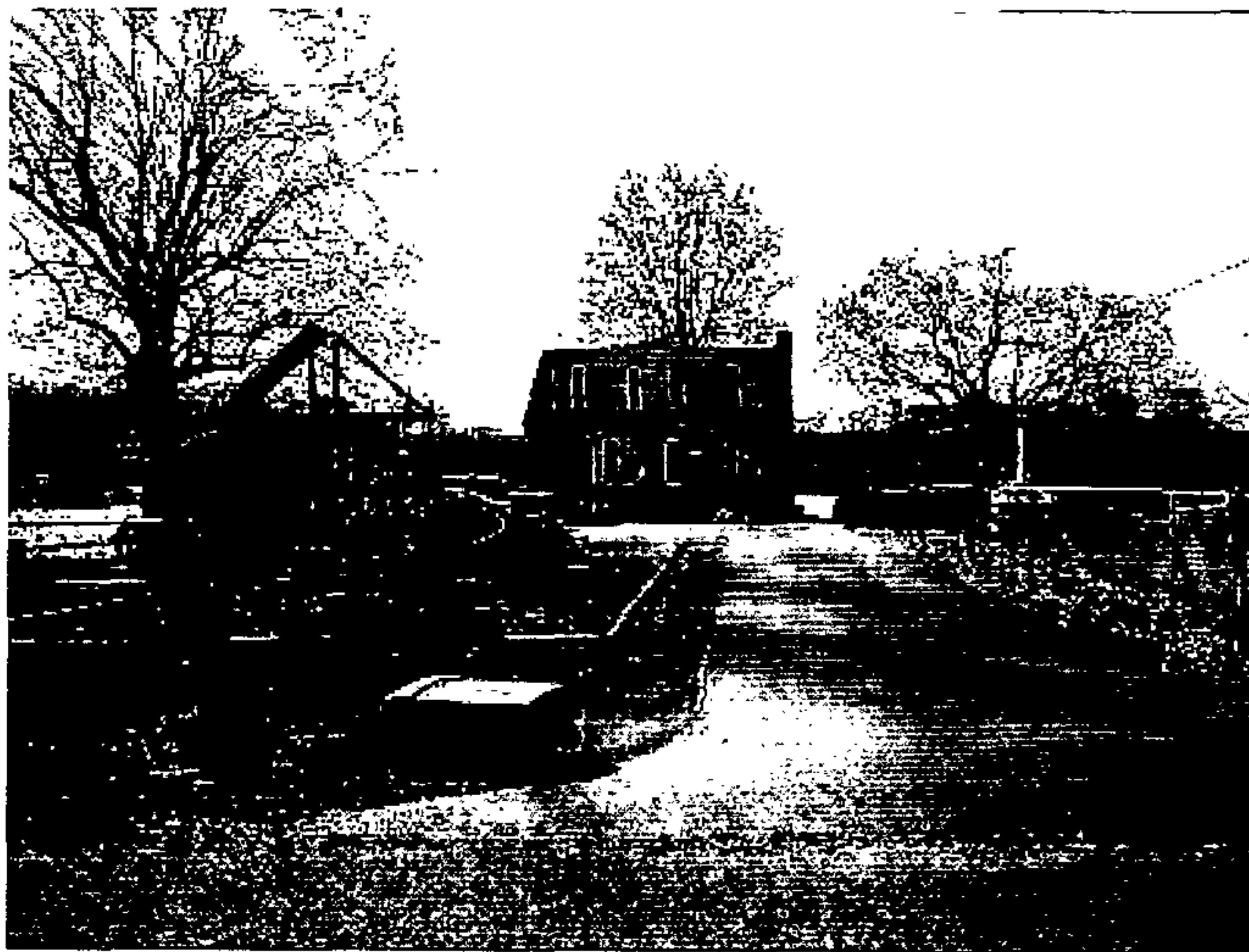
342. WYE RD. (NORTH) STREET SIDE VIEW FROM WYE RD.
