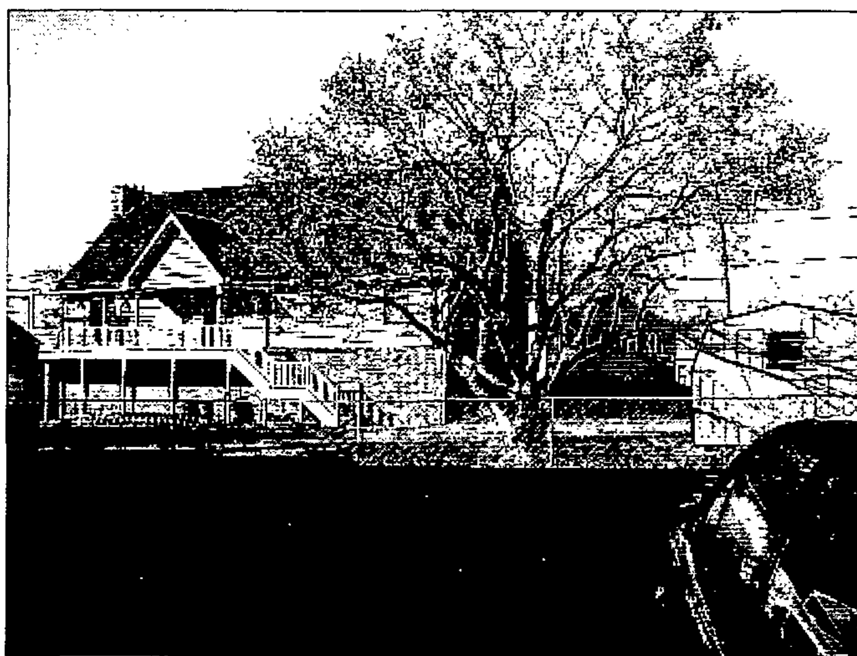
338 WYE RD. (AS FACING 342 WYE RD. PROPERTY)
