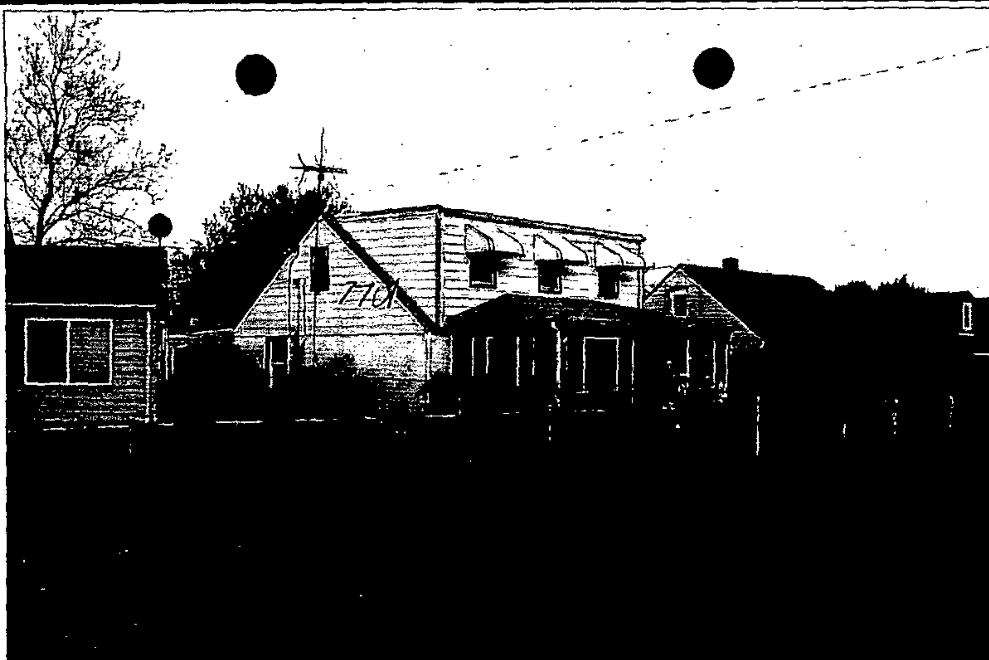
7701 Fair green - 2 nd story and enclosed Porch Addition
