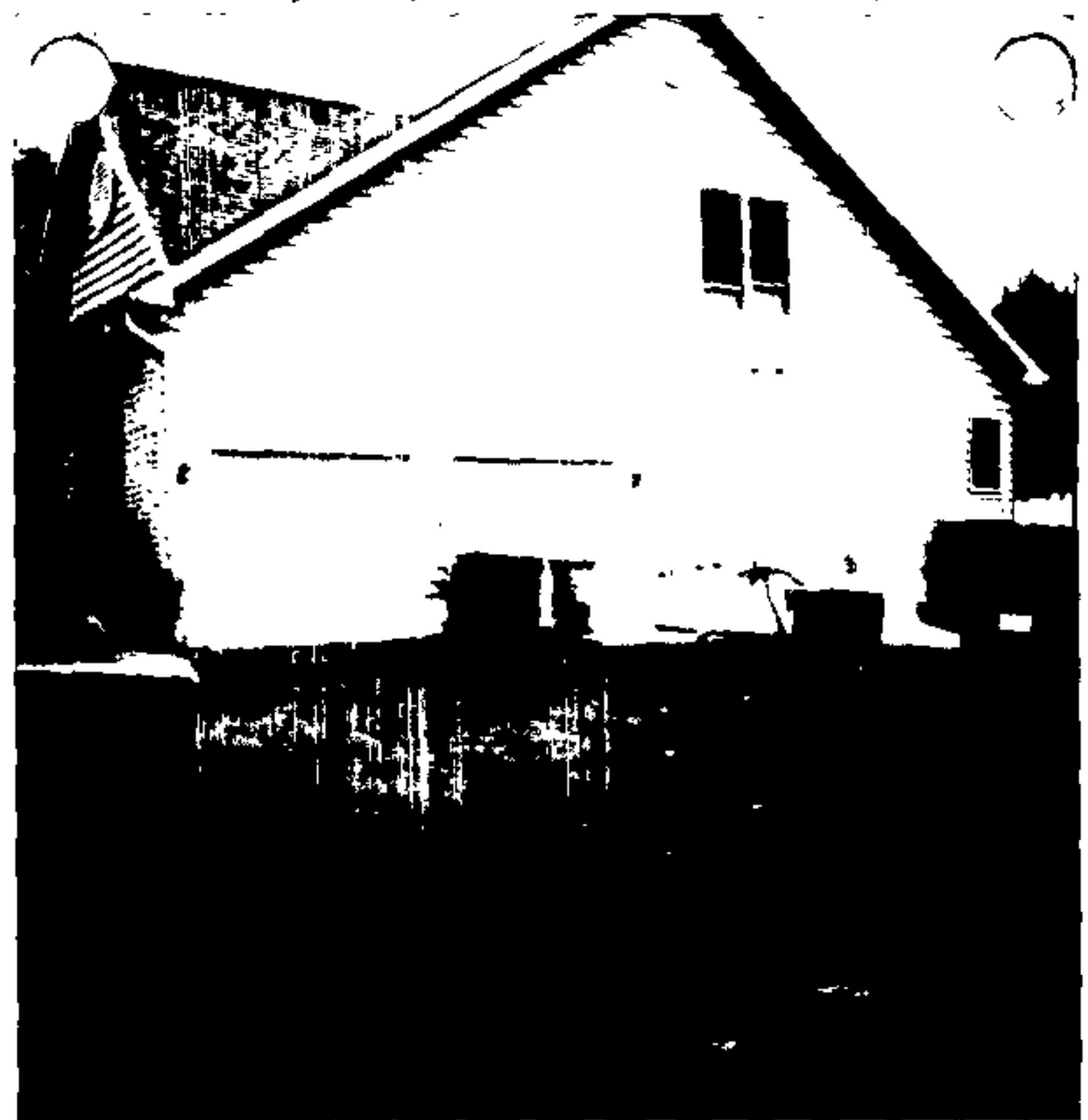
Garage side, area of proposed addition.
