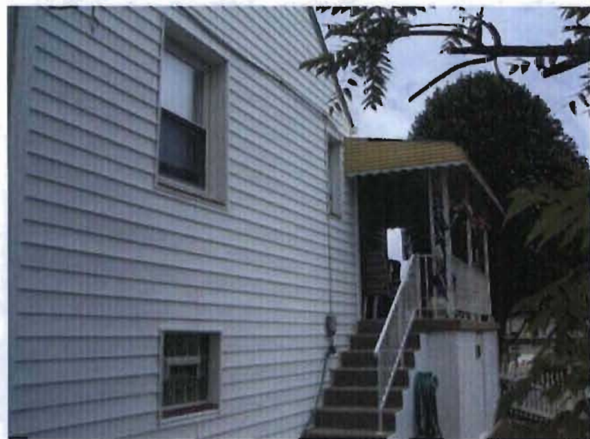
Ext Conc porch on side of house.
