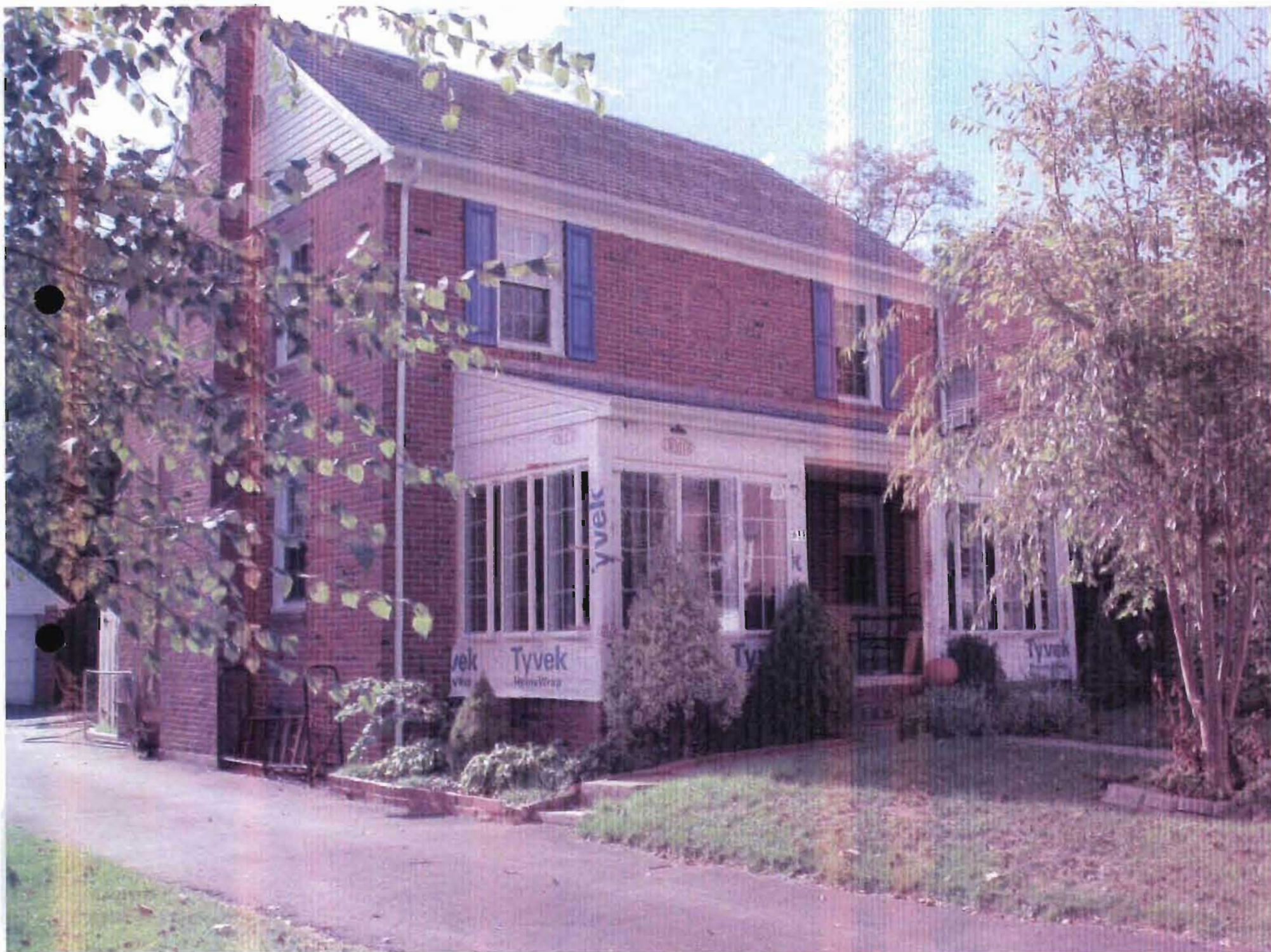
611 Overbrook Road (Left Front)
