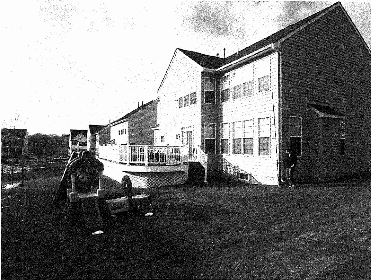
Side View Looking Down Back Yards
